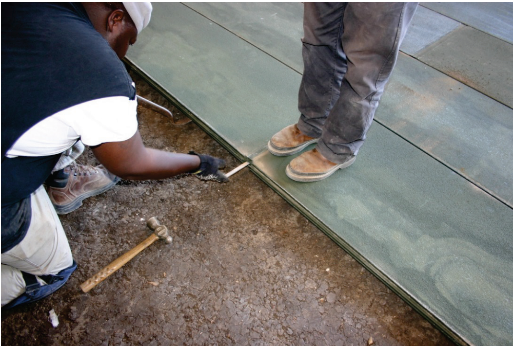
Figure 29. Insertion of AM2 locking bar.
