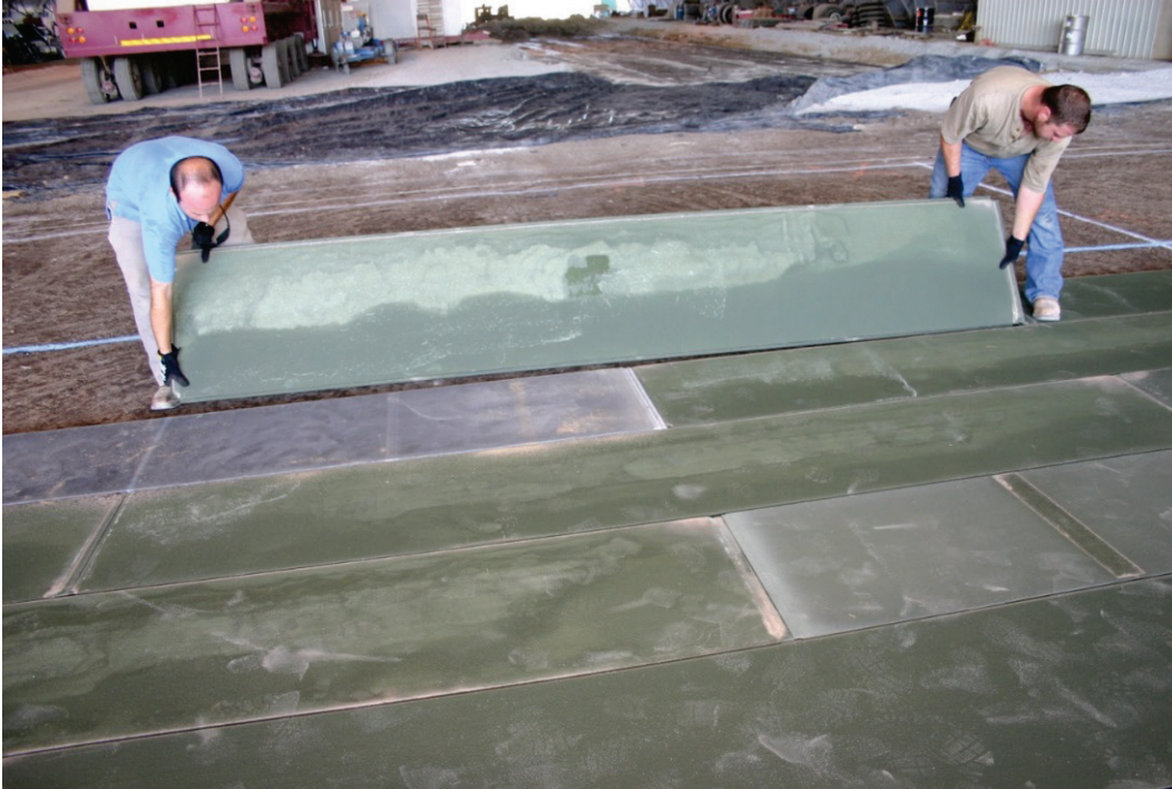
Figure 28. Installation of AM2 panel.
