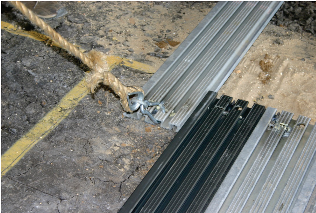
Figure 33. Installation of MLC-70 Trackway panel.
