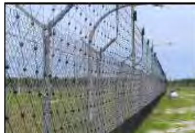
Korean fiber optic mesh detects breaks and enhances perimeter security
