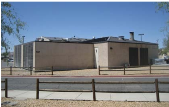
Central Cooling Plant, Bldg. 263 (7th St. off Barstow Rd.)
