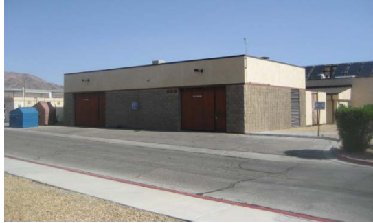
Central Cooling Plant, Bldg. 253 (4th St. off 'B' Ave.) (Chiller mechanical room is on the left side of the building)
