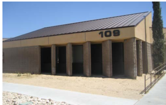
Central Cooling Plant, Bldg. 109 (Langford Lake Rd. off 'B' Ave.) (Mechanical room is at the rear of the building)
