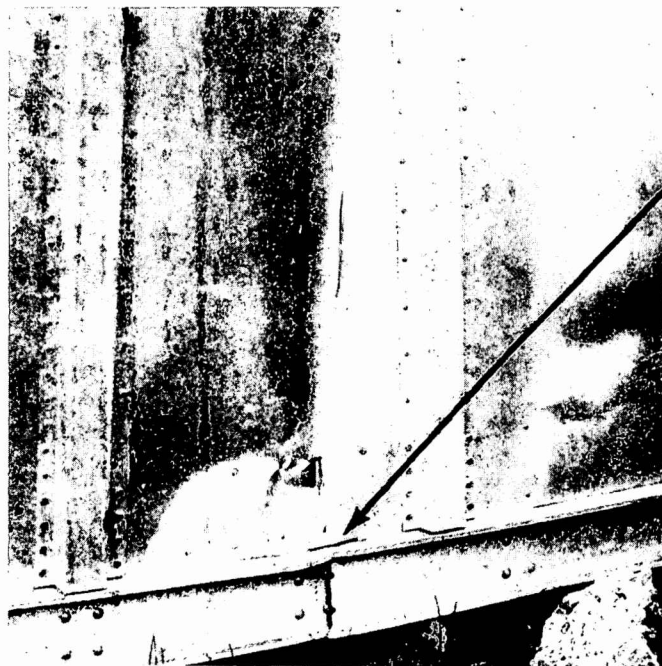
Figure 5-4. Typical Bottom Rail Damage
