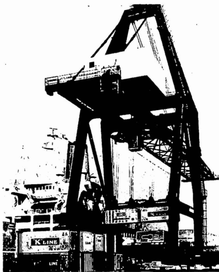
(a) Gantry in Position at Ship's Berth
