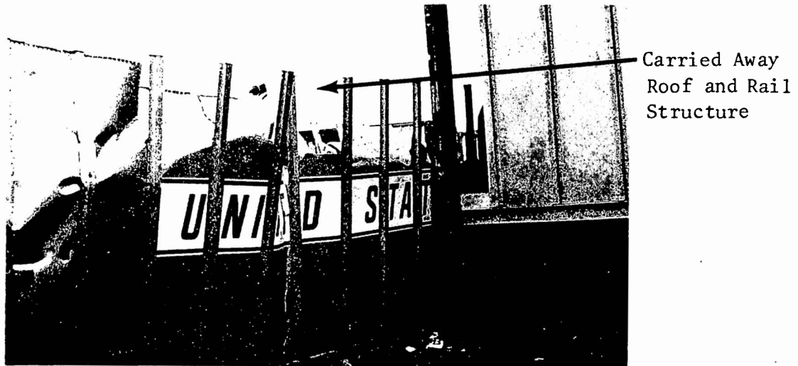
Figure 5-14. Major Roof Damage
