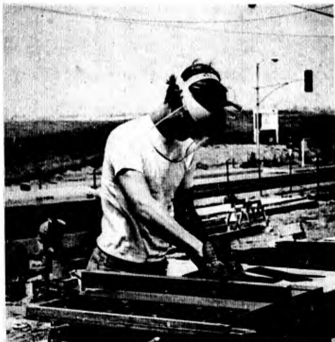
Figure 2-1 Cutting of Reinforcement
