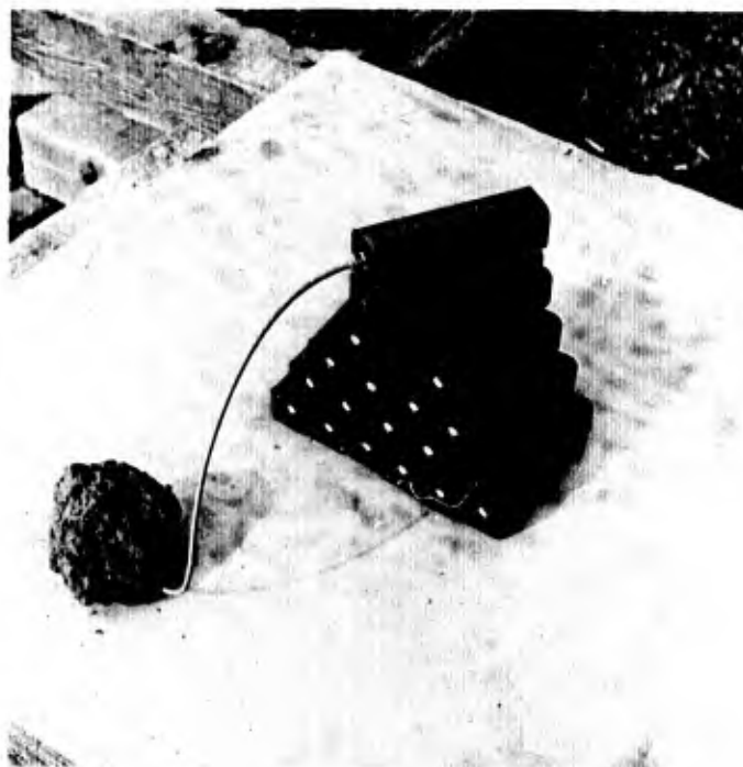
Figure 3-6 Placement of Surface Blast Charge
