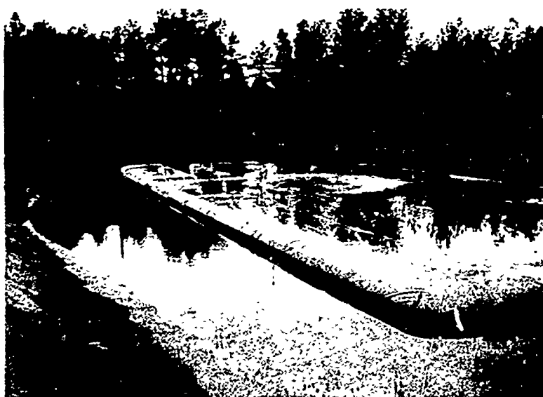
Figure 18. Pooling of water on tank surface; vent pipe submerged.
