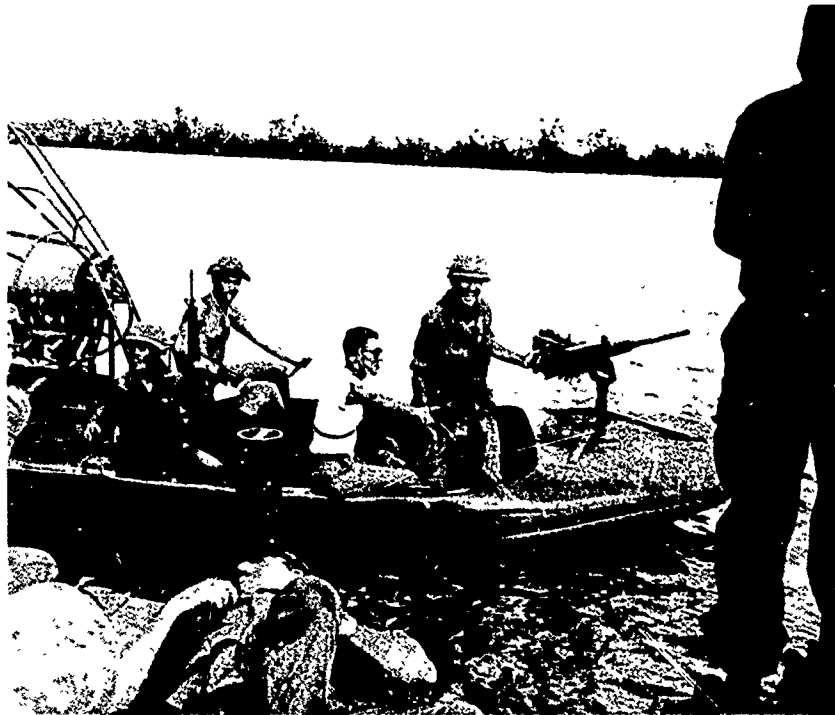
#5 -- Airboat supplied by 15th Engr Bn (C) with Thai security. In addition to providing security, airboats were used to move personnel and supplies to the crushers.
