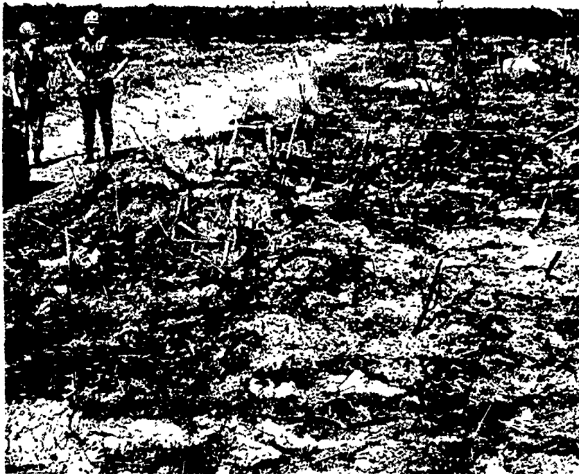
Photograph #6 - (Long Thanh North) Area crushed by transphibian drums further defoliated by burning. Burning took place two weeks after clearing.
