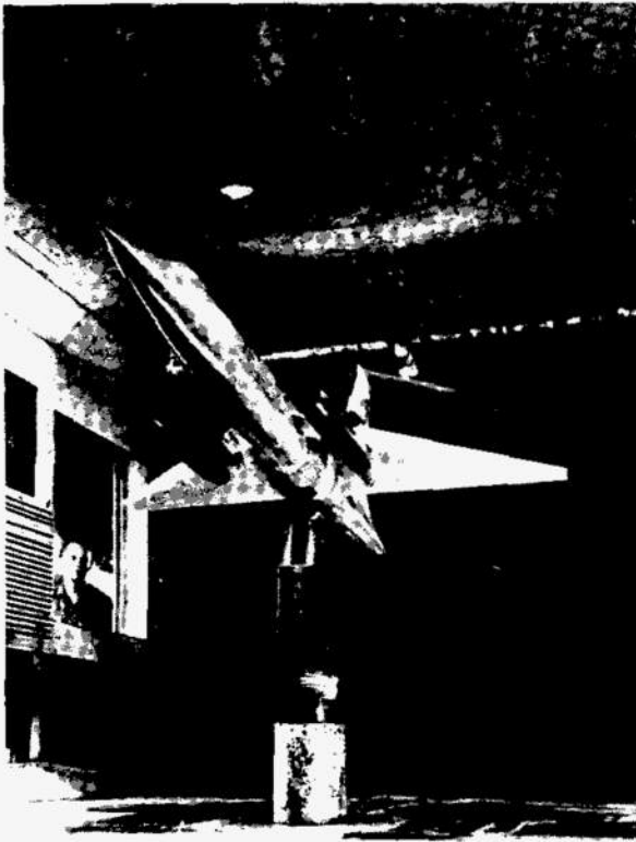
Fig. 4-13 Jet-age aeronautical scientists must assure stability in aircraft over a wide range of speed. Using a high speed research model built for special studies in the 300-mph, 7x10-foot wind tunnel at NACA's Langley Aeronautical Laboratory, scientists evaluate stability characteristics in subsonic flight (e.g., during landing and takeoff) of an aircraft capable of supersonic flight. Automatic recording devices in the adjacent control room measure forces exerted on the test model. The series of spot photographs show the effect of increasing speeds on the shock wave patterns over a supersonic airfoil.
