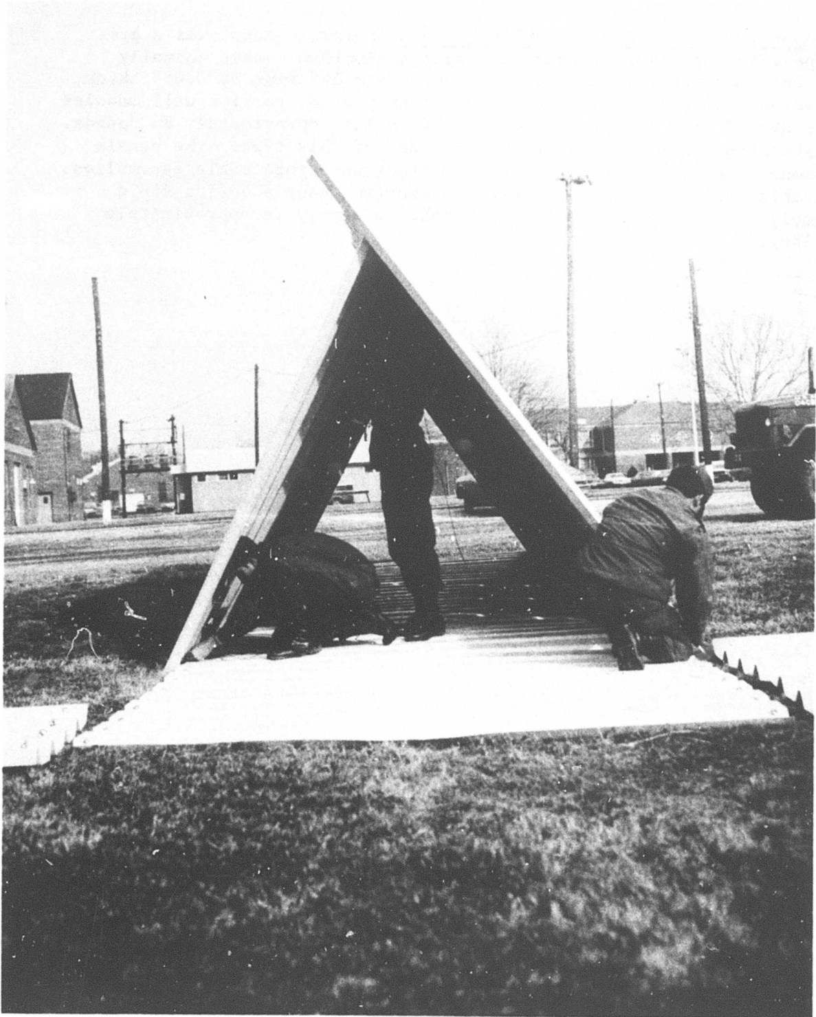
Figure 6. Assembly of Corrugated Aluminum Panels Using Wire Cables for Fastening.
