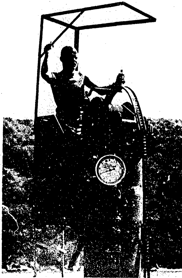
Fig. B51 - Tensionometer in use to control the descent of the launch barge
