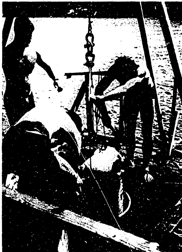
Fig. B3 - Canister for dry transfer between the surface and the habitat
