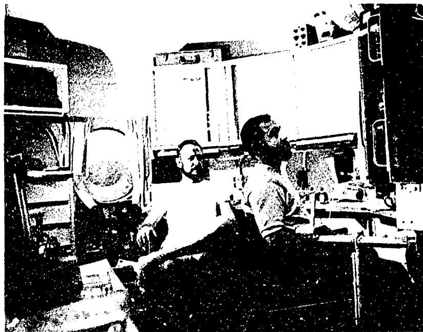
Fig. 20 - Aquanauts Van Derwalker and Waller checking the habitat systems on the bridge of the habitat. Note the psychomotor test device at the lower right and the emergency escape bottles under the circular port to the left
