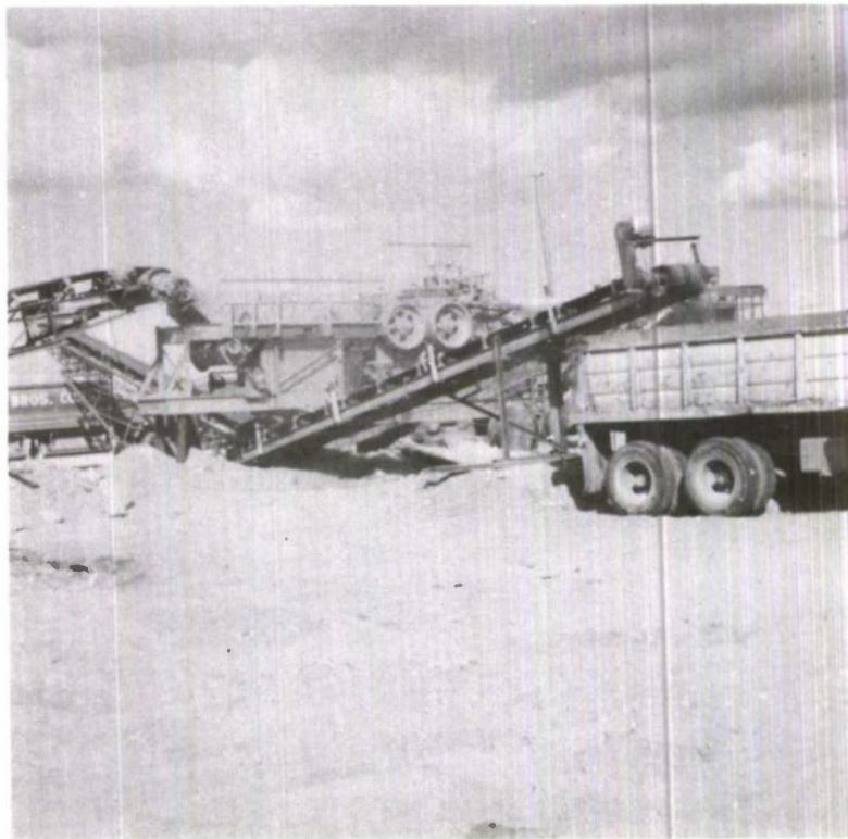
Figure 2.7 Sieving of ejecta from the Mineral Rock crater lip at a rock-crushing plant (Western Rock Products Corp., Cedar City, Utah).
