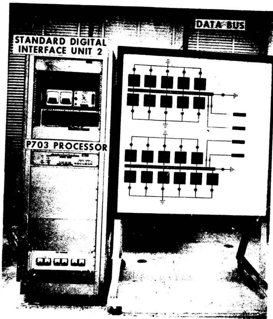
Fig.7 Electrical power subsystem/processor and panel
