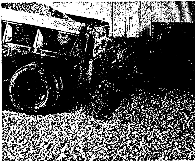
Fig. 3. End-dumping of rock in item 3'
