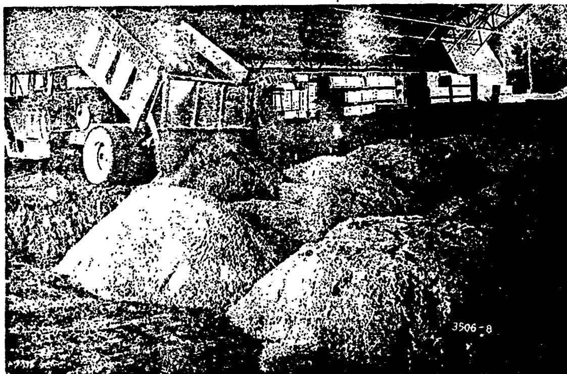
Fig. 4. End-dumping of sand in item 4
