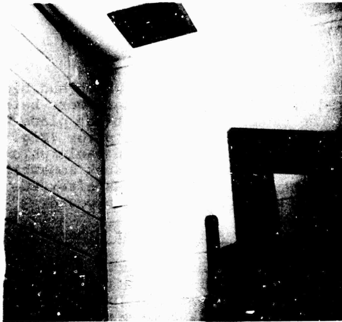
Fig. 1 An old crack has opened up in the Station Chief's office at the ORC Station 6 months after redecoration.
