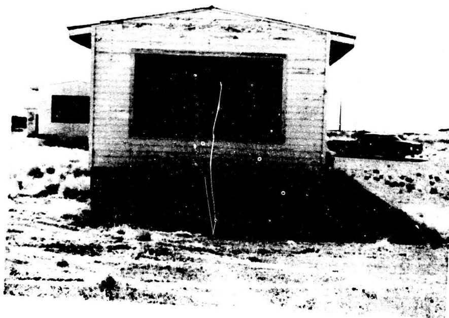
Fig. 28 W-4, Northerly exterior
