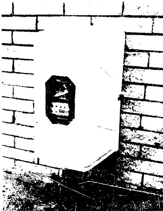
Figure 9. Outdoor Meter and Regulator Set Enclosed in Plastic Case.
