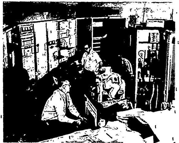
Instrumentation associated with the tower vacuum telescope is placed on a platform that revolves in carousel fashion as the optical system rotates to follow the sun.
