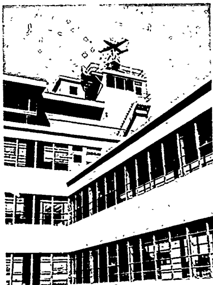
This model of a C-121 was placed at the highest point atop AFCRL's main laboratory complex for tests of the SAD-FRAD radar antenna (wavelengths were scaled correspondingly) prior to the design of the antenna system.
