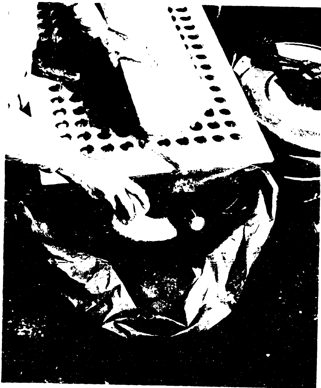
Figure 10. Asbestos refuse collected in polyvinyl plastic bags are sealed and removed from the ship. This reduces a major source of asbestos dust and simplifies clean-up.
