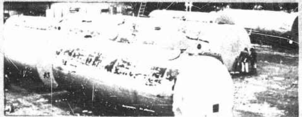
Fuel tanks in hangar being modified for ice containers.
