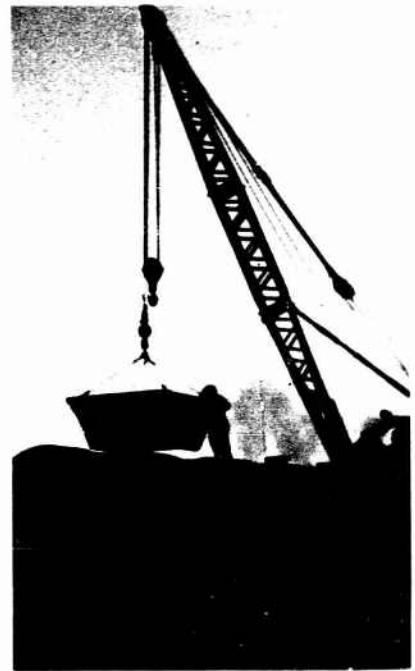
Crane lowering a chule into 25,000-gallon tank preparatory to loading it with contaminated snow and ice.
