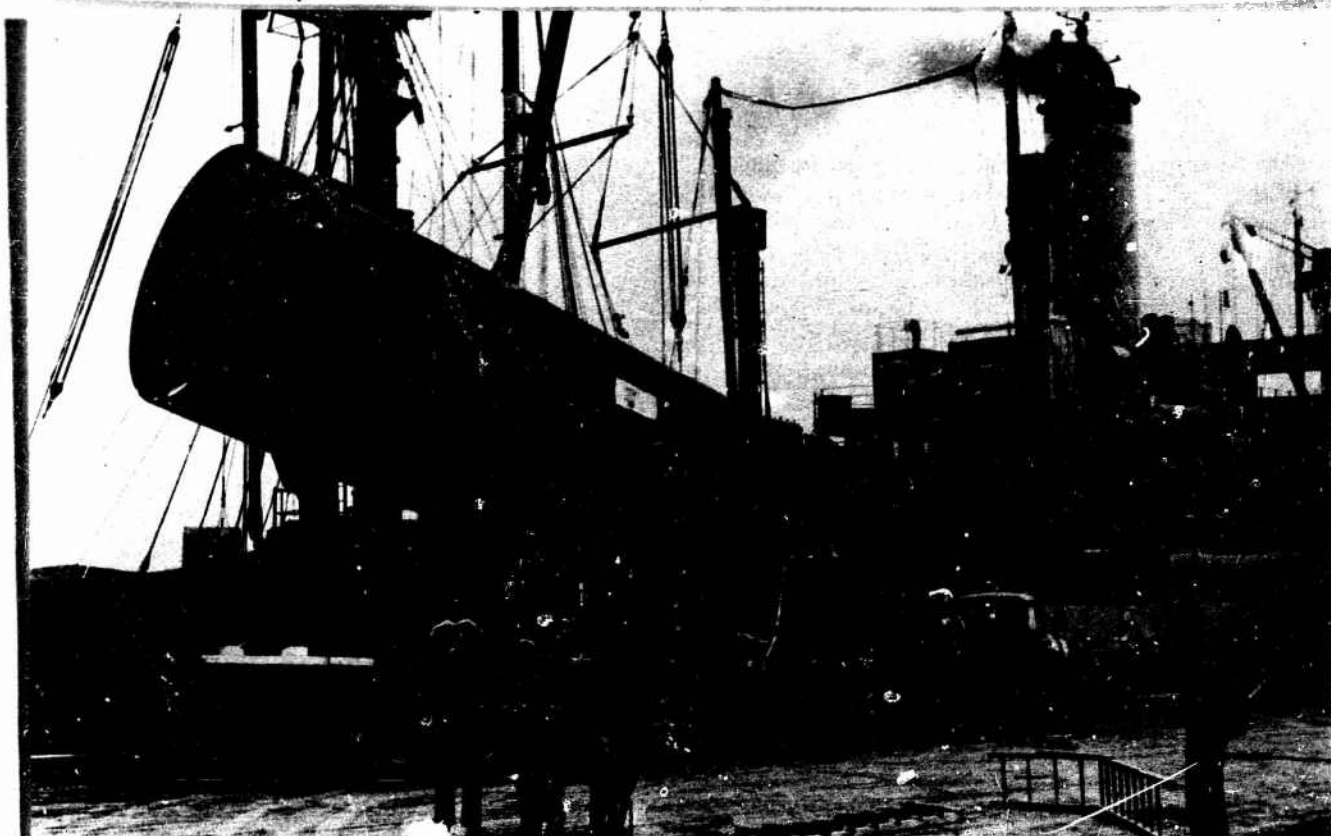
Fuel tank being lifted onto floe by crane.
