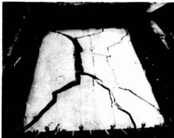
c. 1584 psf ( 7733.8 \text{ kg/m}^2 ), failure
