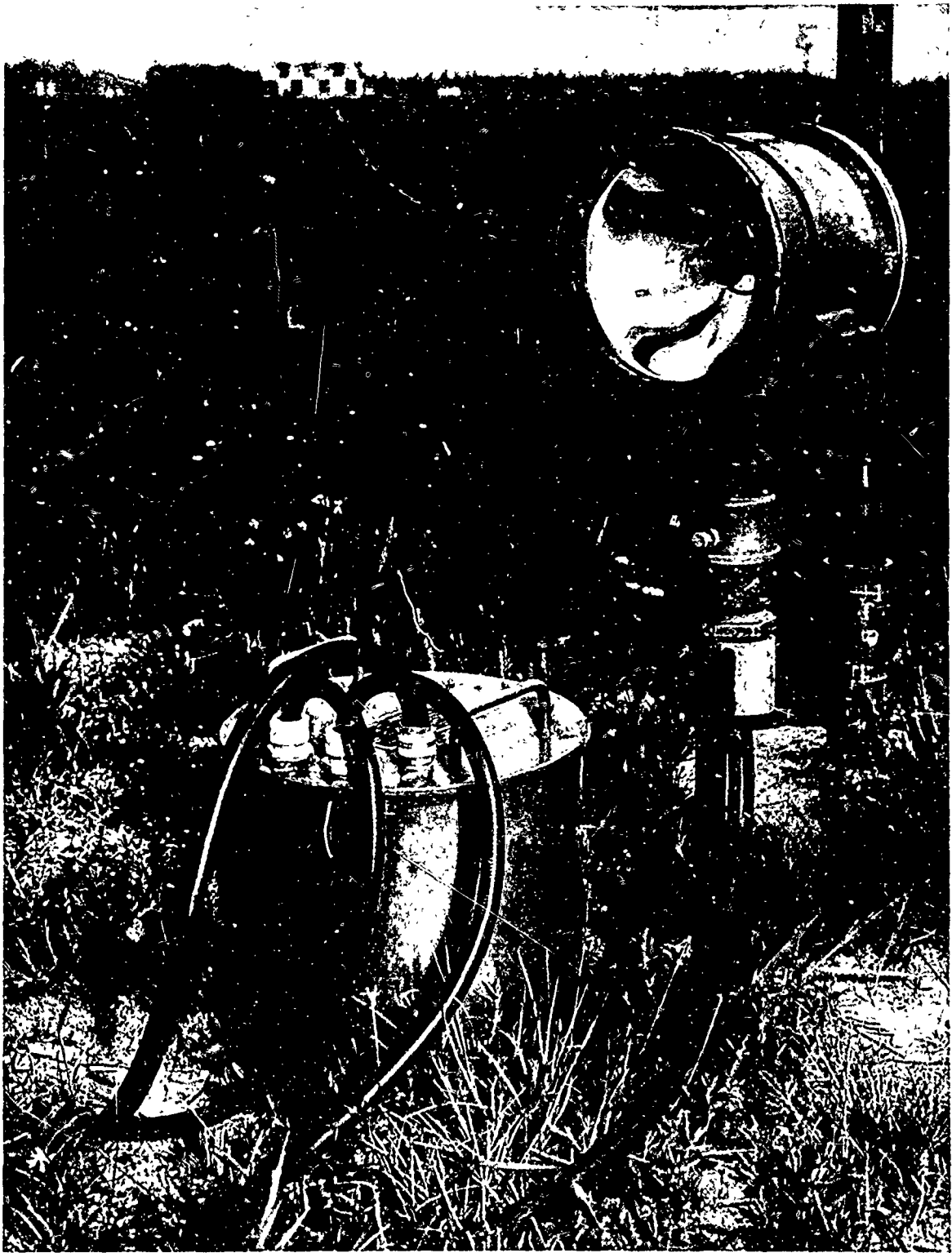
FIG. 3 TYPE FAA-1250 CONDENSER-DISCHARGE STROBE LIGHT
