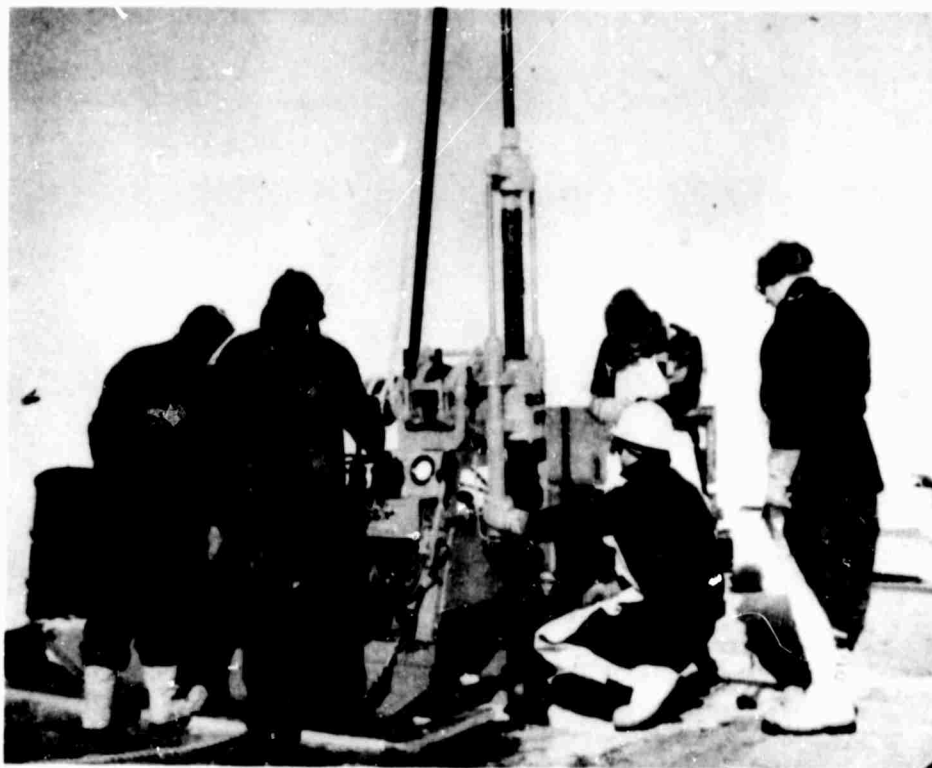
Drill rig showing large diameter coring auger in use.
