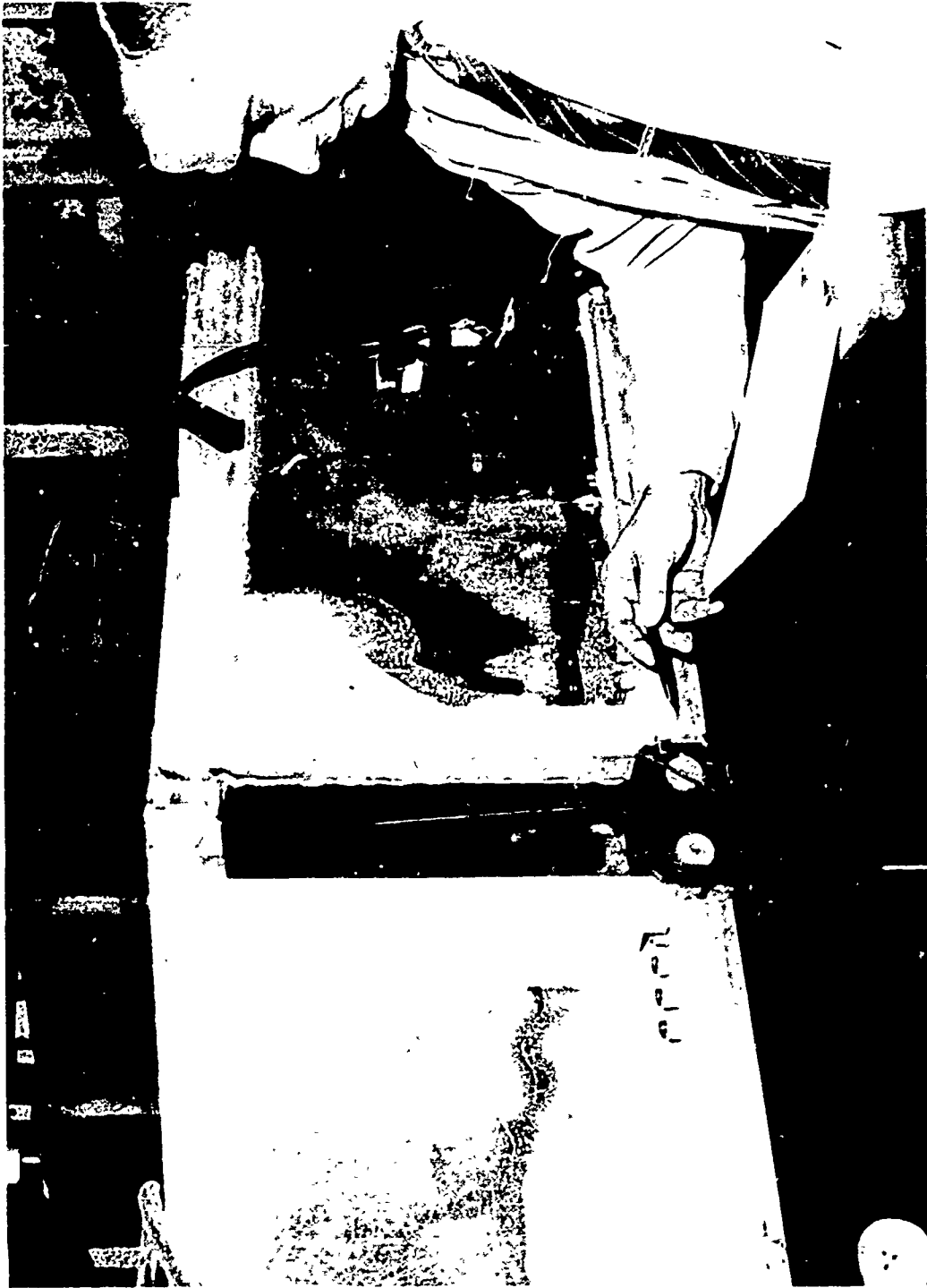
Fig. 3. Two-centered, noneccentric hinge.
