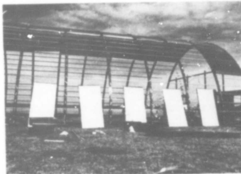
FIGURE #26 - Wood beams and plywood sheathing - Live Structures, Inc.
