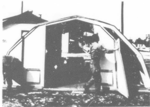
FIGURE #14 - Field Erection of 16'x16' test shelter
