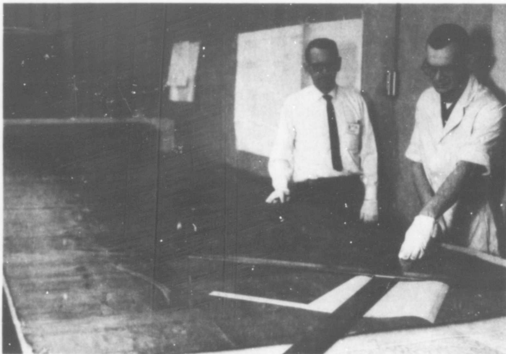
Figure 4. Layout and Cutting of Fabric
