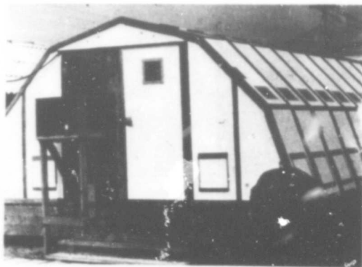
FIGURE #12 - Air Conditioning unit in improved shelter, Vietnam, Summer 1966.
