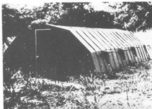
FIGURE #6 - Shelter in jungle clearing test site- Howard AFB, Canal Zone, October 1965
