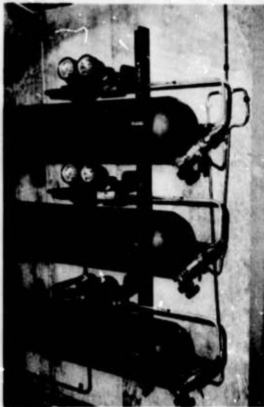
Fig. 5. Compressor room regulators and receivers
