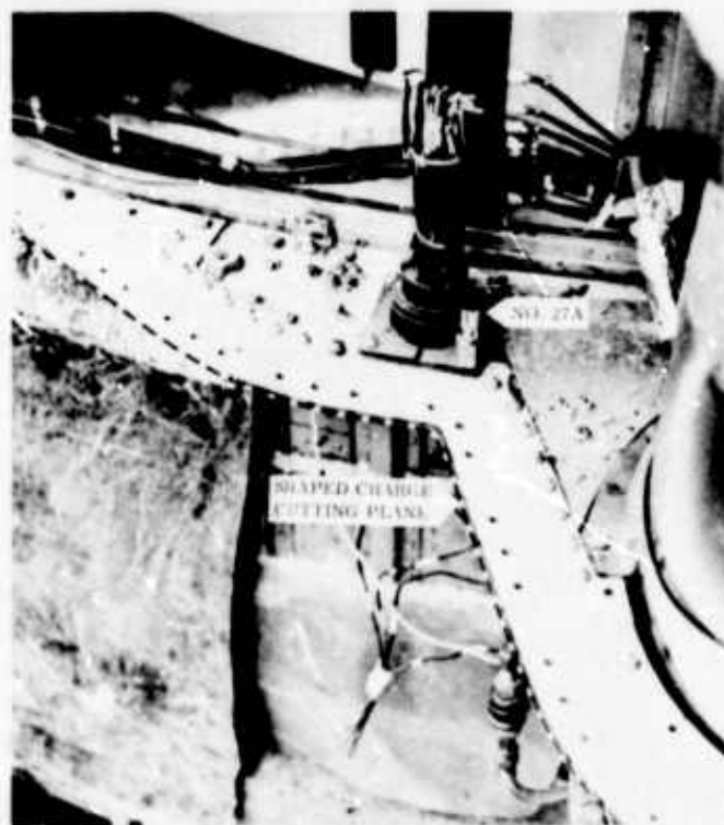
Fig. 6. Accelerometer on electrical wiring staging disconnect
