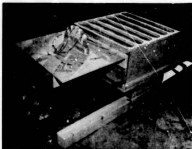
Fig. 6. Typical wooden chamber explosive test setup
