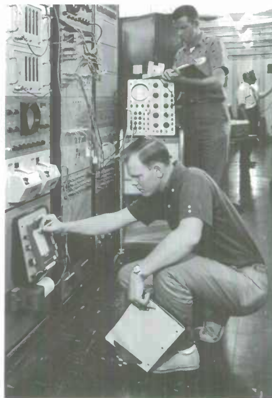
This receiving and data measuring equipment was used at Riverhead, New York, during two 30-day tests to determine the effects of high-frequency propagation on digital data transmission.
