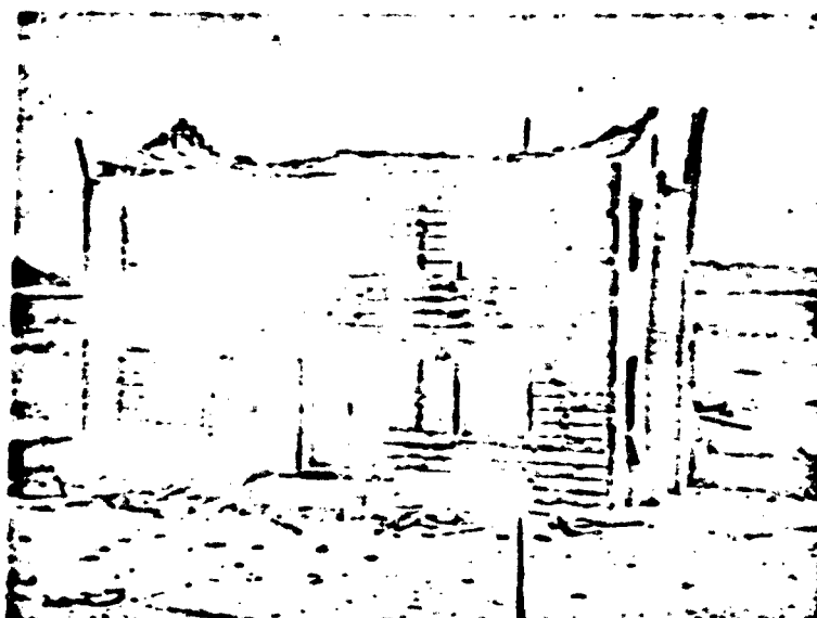
FIGURE 4. Strengthened Wood-Frame House Exposed to 4 psi Overpressure and About 25 \text{ cal/cm}^2 Thermal Energy (5,500 feet from 29-KT Burst on a 500-ft Tower)
