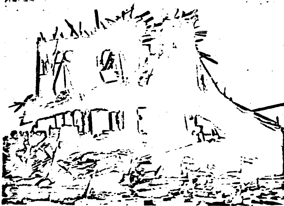
FIGURE 5. Unreinforced Brick House Exposed to 5 psi Overpressure (4,700 feet from 29-KT Burst on a 500-ft Tower)
