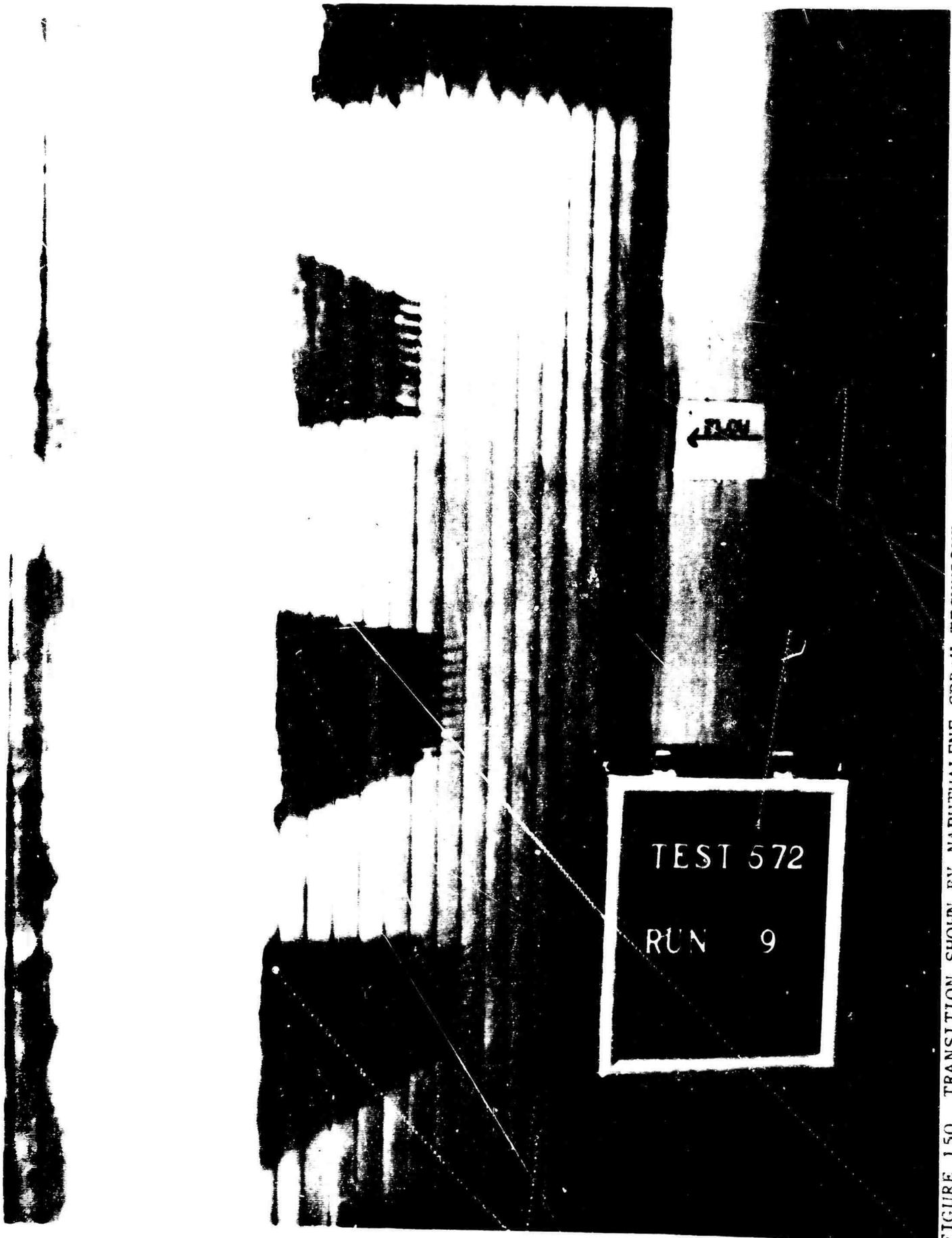
FIGURE 150 TRANSITION SHOWN BY NAPHTHALENE SPRAY TECHNIQUE. INTERNAL SOUND. 150 DB. 582 CPS
