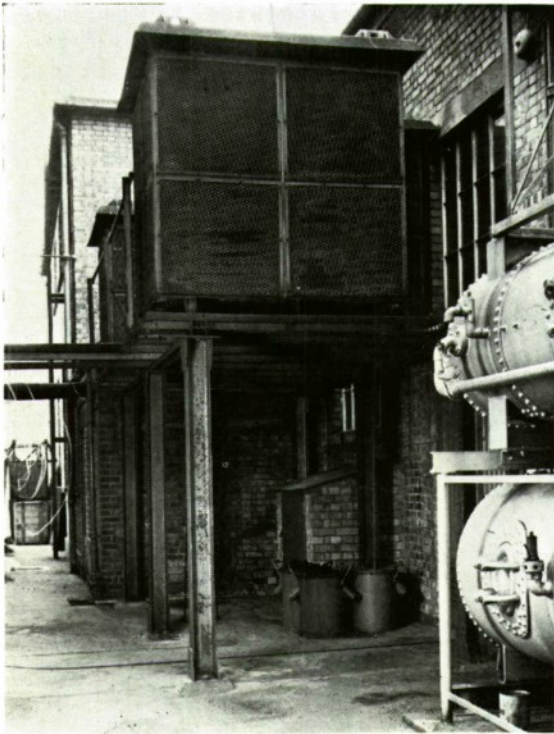
FIG. 4. 350 kW Resistance Load Bank for Paxman YHA Diesel Engine.
