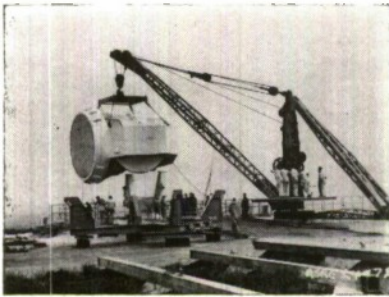
The 3D Radar Aerial being installed at ASRE in 1953 in the new "3D Radar Building". This was the first experimental radar fitted at ASRE, Portsmouth.
