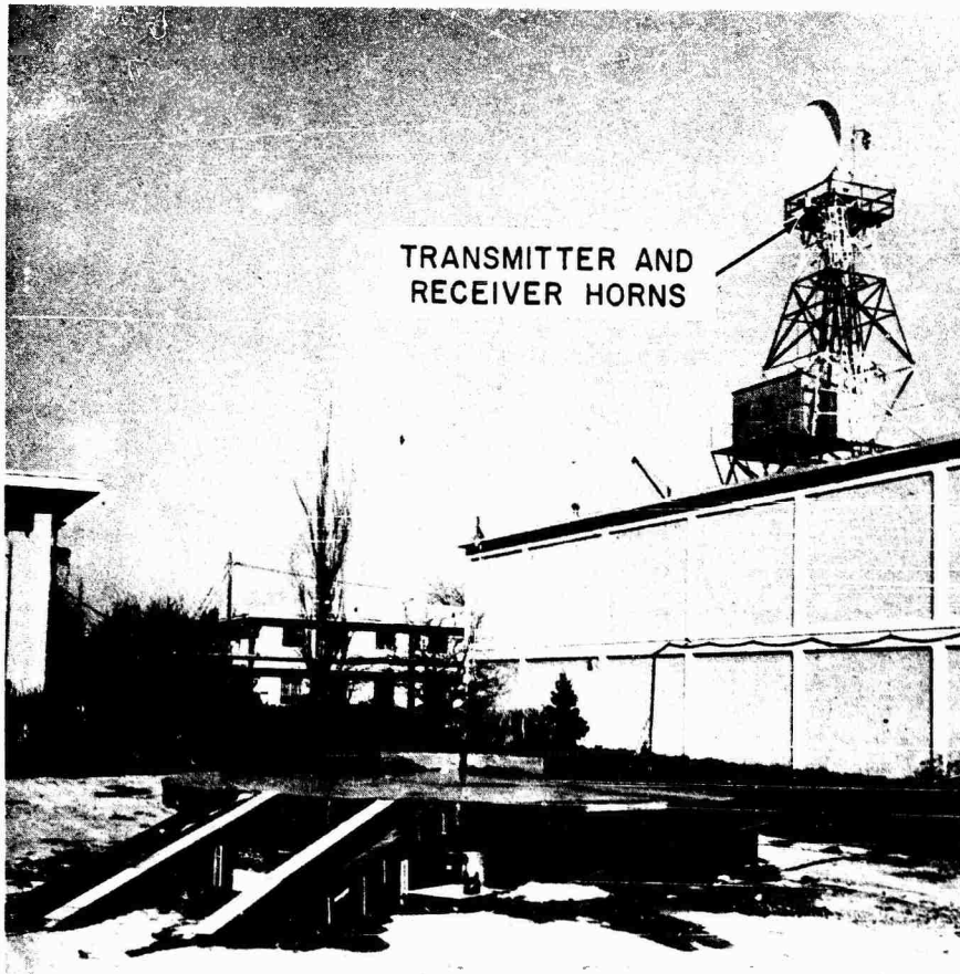
FIGURE 9. ROTATING PLATFORM RADAR FACILITY
