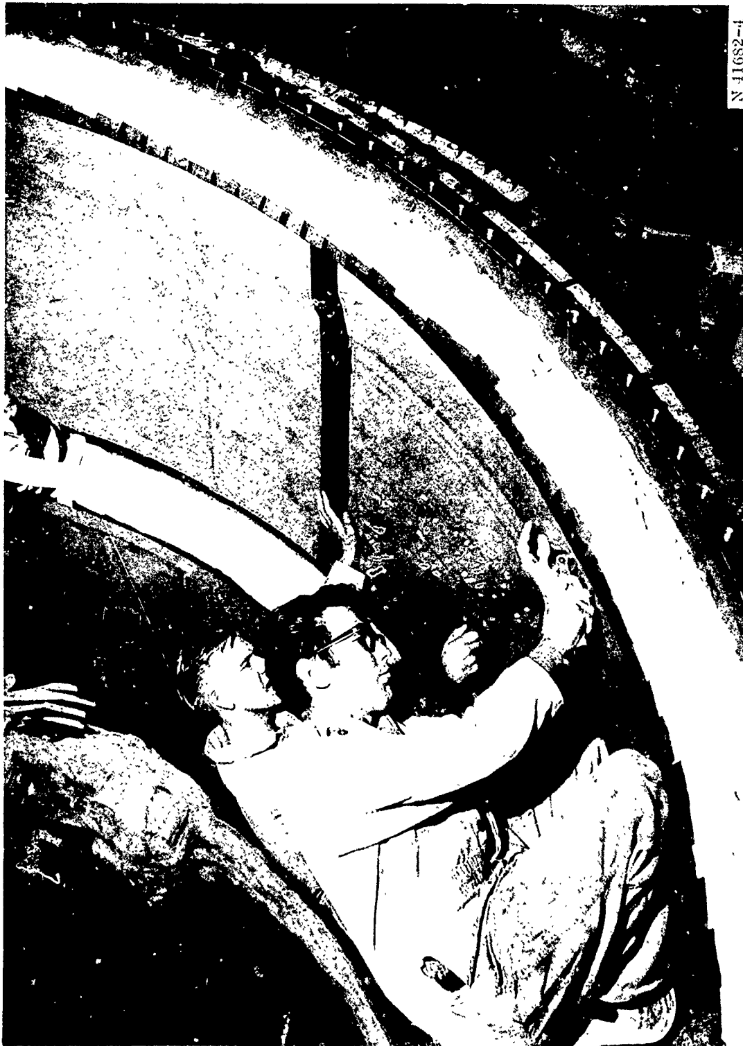
Figure 50. Rolling and Stitching V-44 Sheets for Laminate
