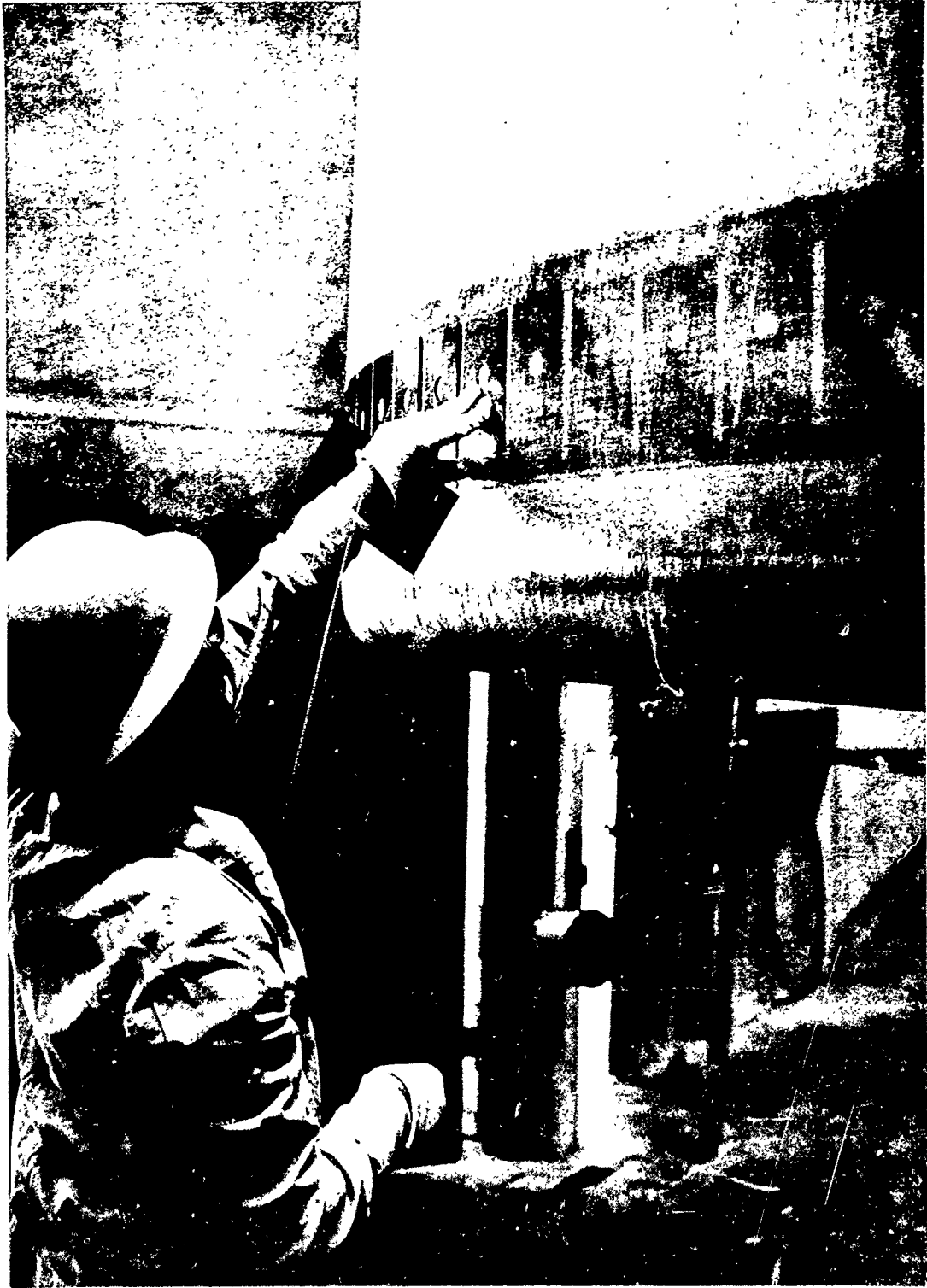
(U) Figure 10. Shim Placement
