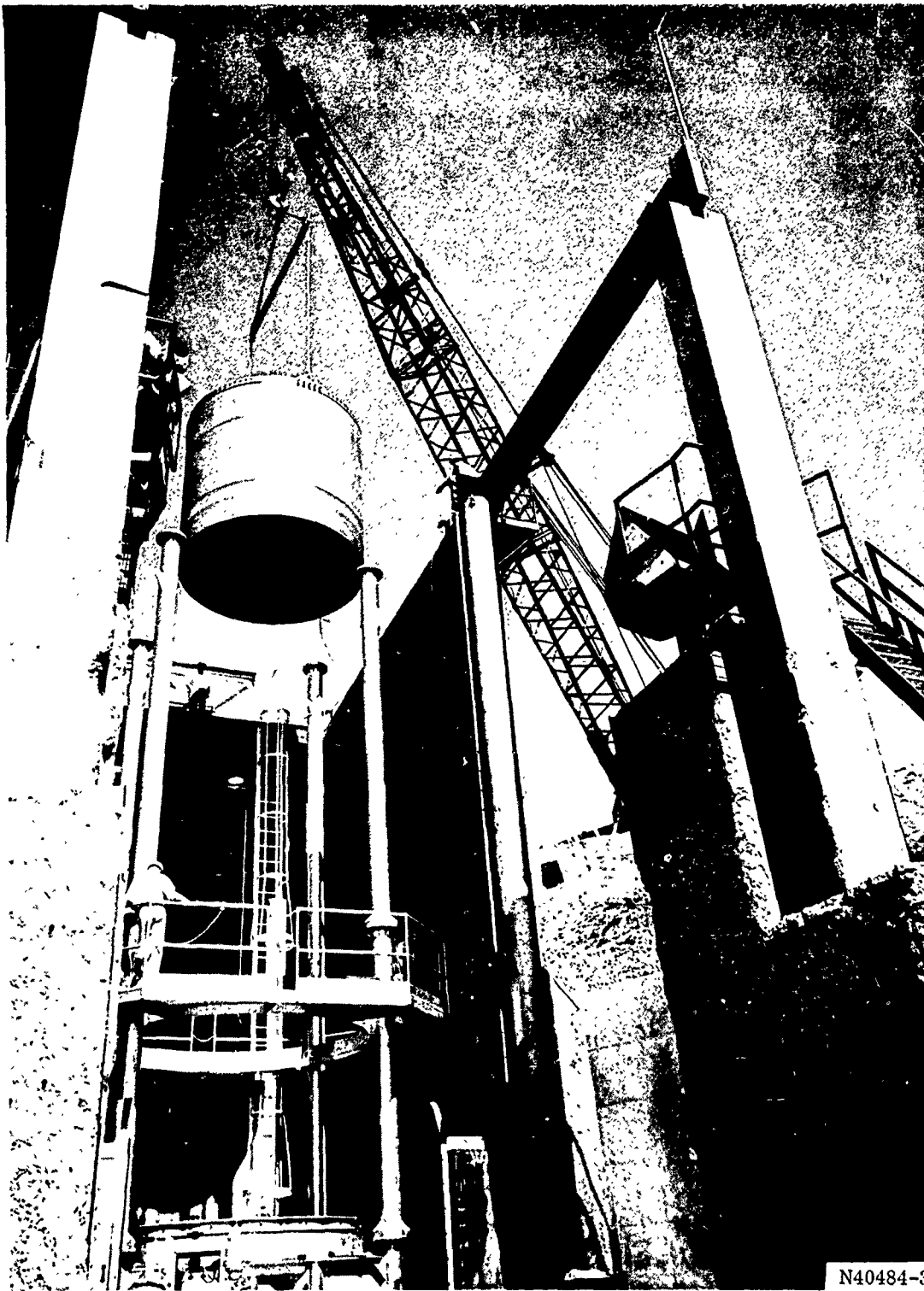
(U) Figure 70. Lowering Forward Segment into Place
