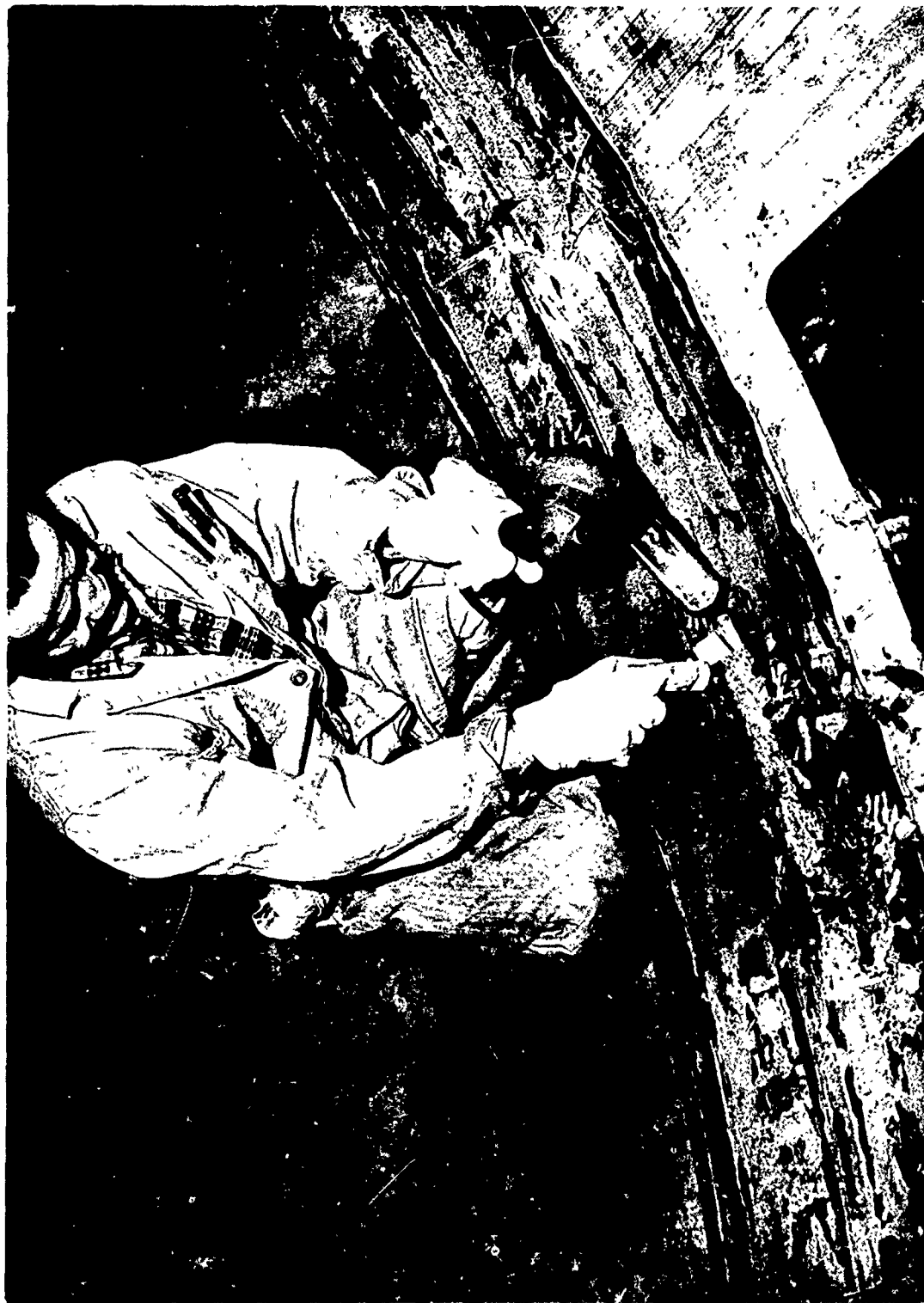
(U) Figure 14. Removal of Buna-N Strips from Joint Areas
