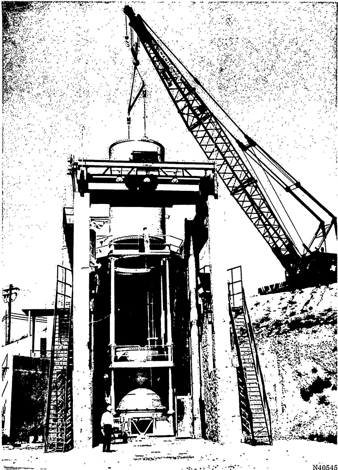
(U) Figure 72. Lowering Center Segment into Place
