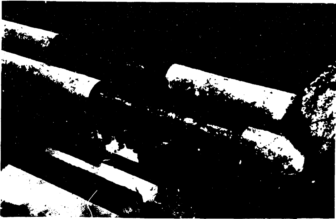
Figure E-1. Seattle. The insulation has been removed from the pipe revealing that both pipe and insulation are in aood condition.
