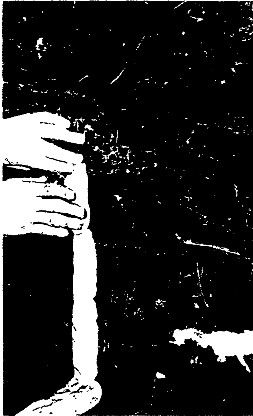
Fig. 25. Hand placement of paste explosive on to grease-coated steel beam.
