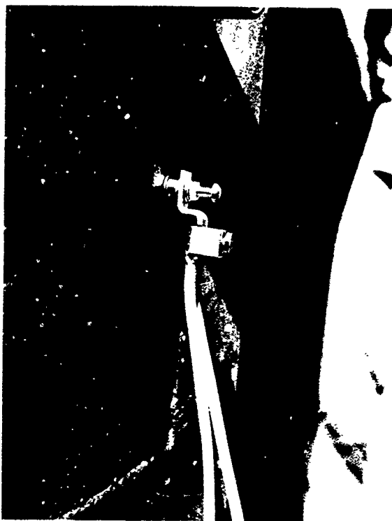
Figure 19. Ground Connection
