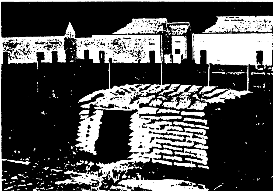
Figure 4. Rectangular Shelter Before Installation Within the Test Structure
