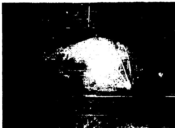
Fig. 10. The air-supported structure fully inflated and ready for the spraying operations. The plastic membrane consists of nylon mesh with an inner facing of Mylar and an outer facing of polyethylene.
