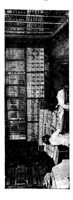
Fig. 1—The "Strela" electronic calculating machine
