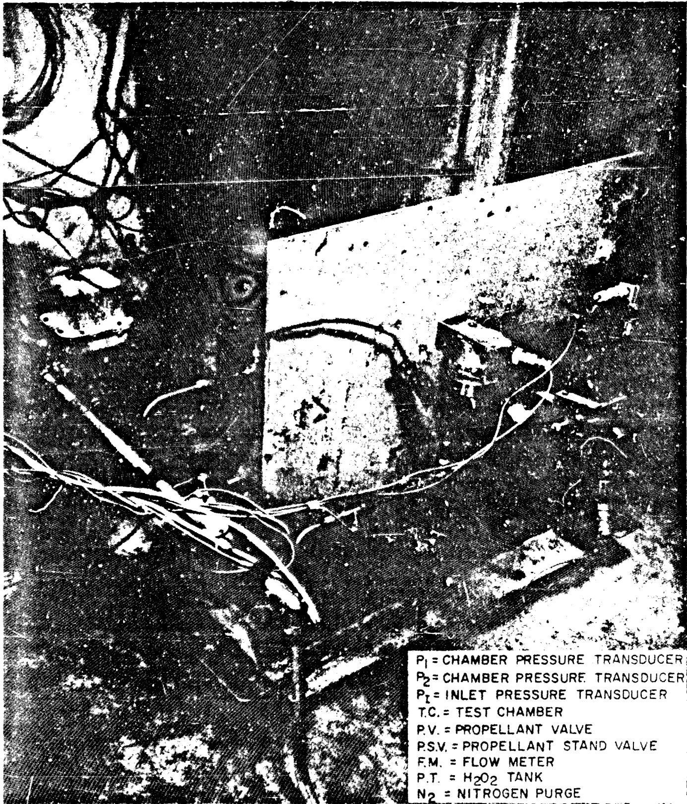
HIGH PRESSURE TEST STAND AT WALTER KIDDE COMPANY
