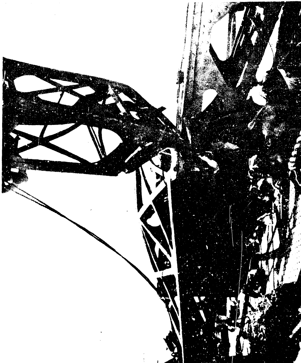
Airplane crane, USS NEVADA after Test VBLE. Lower leg of the crane bent over the stern of the catapult starboard side.
