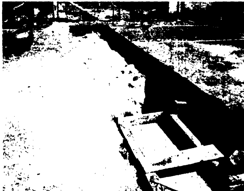
Figure 9. The trench is backfilled with sand.
