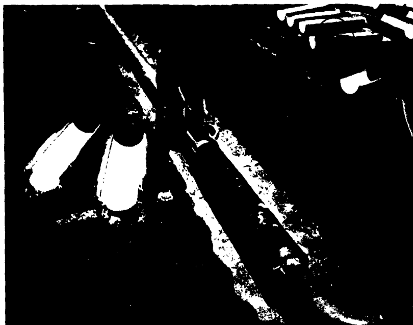
Figure 5. Installing the Foamglas inculation.
