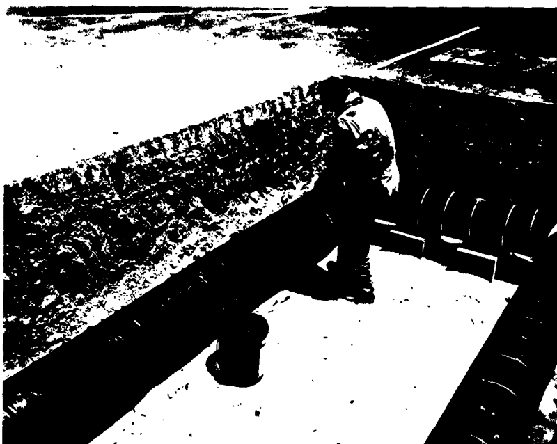
Figure 13. Sealkote being applied to loop piping.
