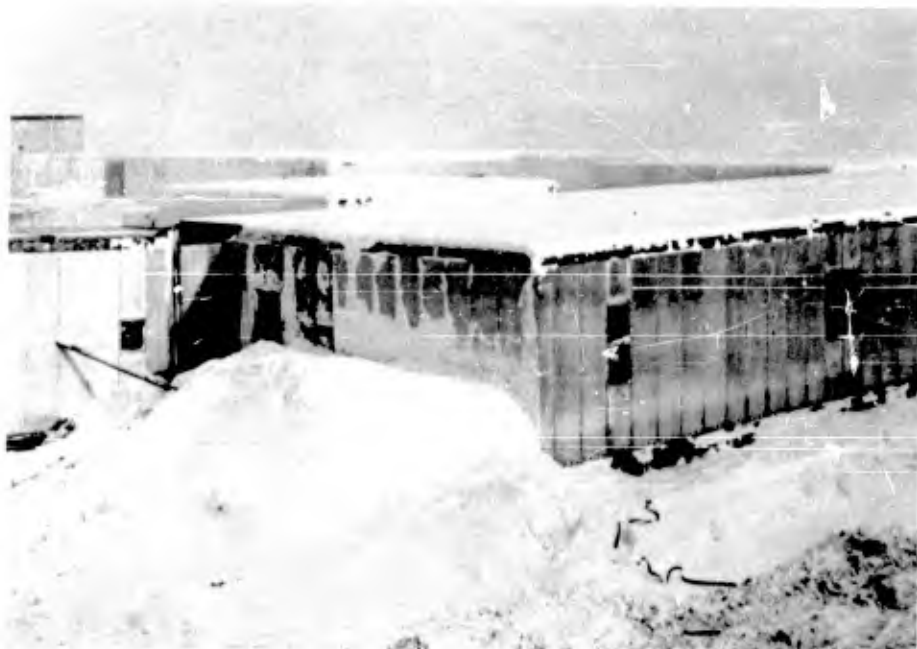
Figure 26. Thule barracks area in April. These buildings were erected on blocks three to four feet above the ground surface.
