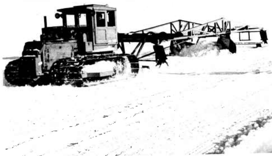
Figure 14. Modified land plane used on Greenland Ice Cap in 1954 to plane snow runway.
