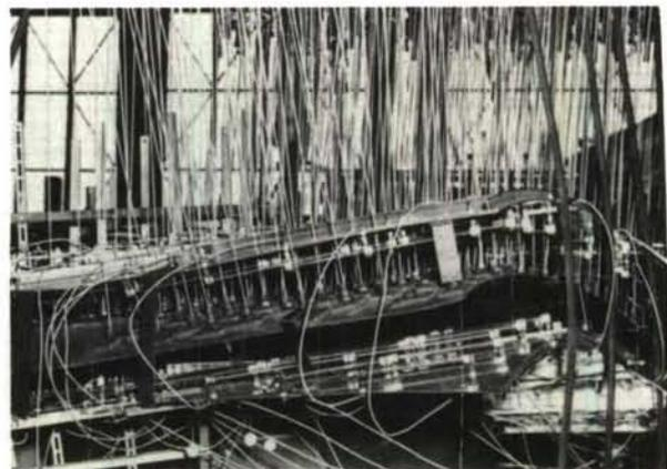
Figure 3A and 3B. B-58 Wing Tip Elevated Temperature Test Using RTV Silicone Bonded Tension Patches
