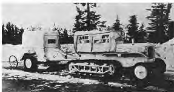
FIGURE 41. T-26 snow tractor with trailer (on wheels) equipped with odograph. (Note odometer wheel behind trailer.)
