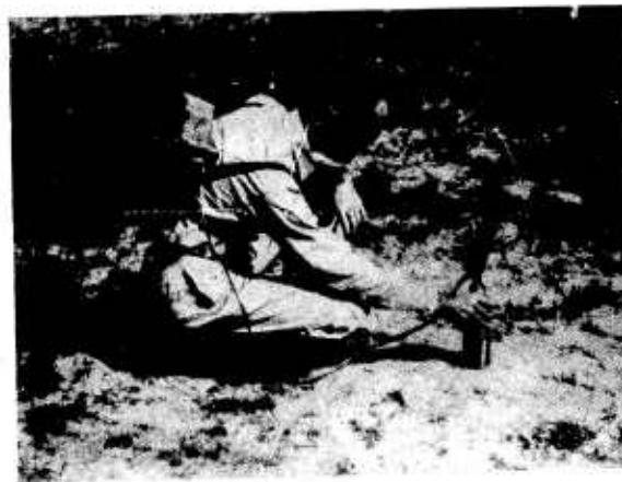
FIGURE 20. Prototype instrument as adapted for use when crawling.
