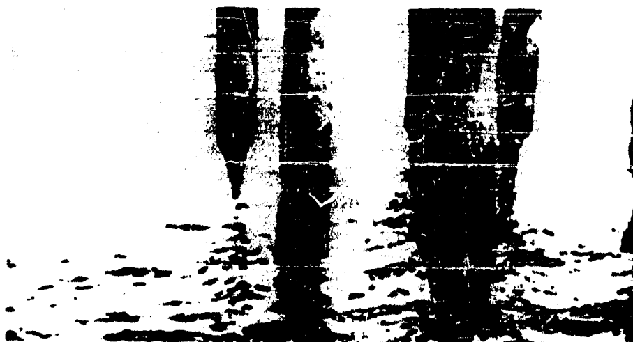
Figure 18. Piling Destroyed by Limnoria
