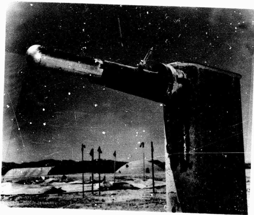
Figure 2.34 IRL dynamic-pressure gage adapted to standard AFSP mount.
