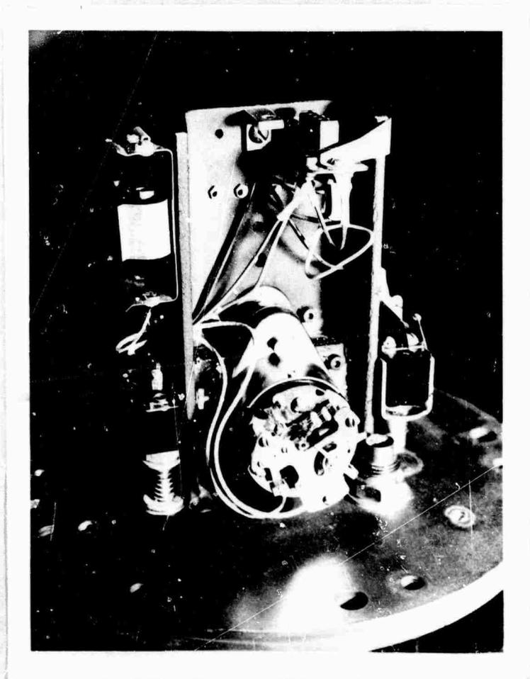
Figure 2.3 Disk-drive motor for self-recording gage.
