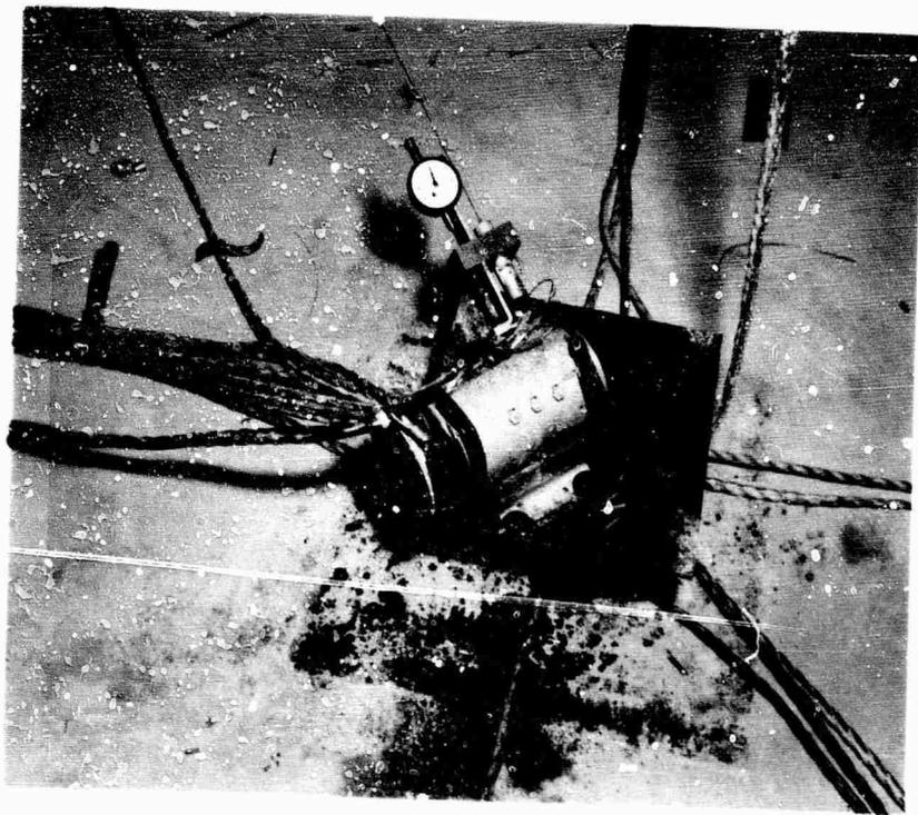
Figure 2.40 Small-displacement gage calibration.
