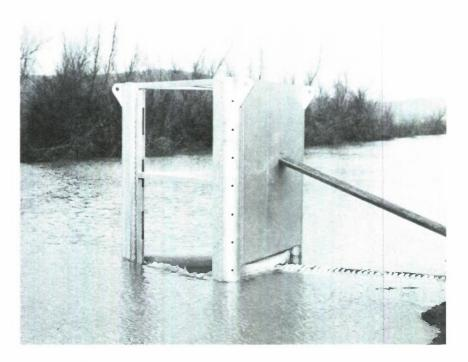
Effluent leaving disposal area through spill box at disposal area south of Rio Vista
