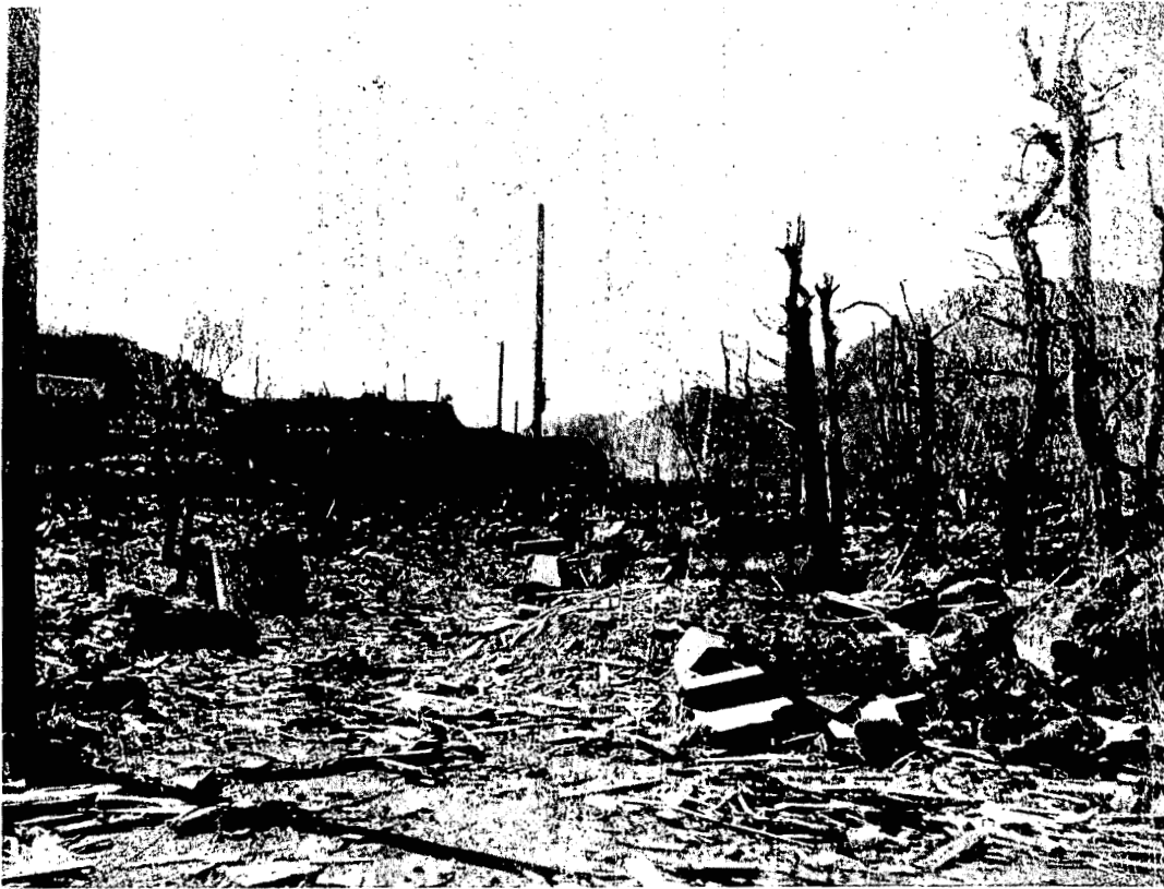
Fig. 9 (5N)--Yamazatomachi, a residential section, just beneath the point where the bomb exploded. Notice that the trees and poles are standing, but with branches and cross-arms stripped off. The complete demolition of houses is shown. Notice that all the debris did not burn. There are no known survivors from this district except people who were inside cave-shelters. (Photo File #NG 168.)
