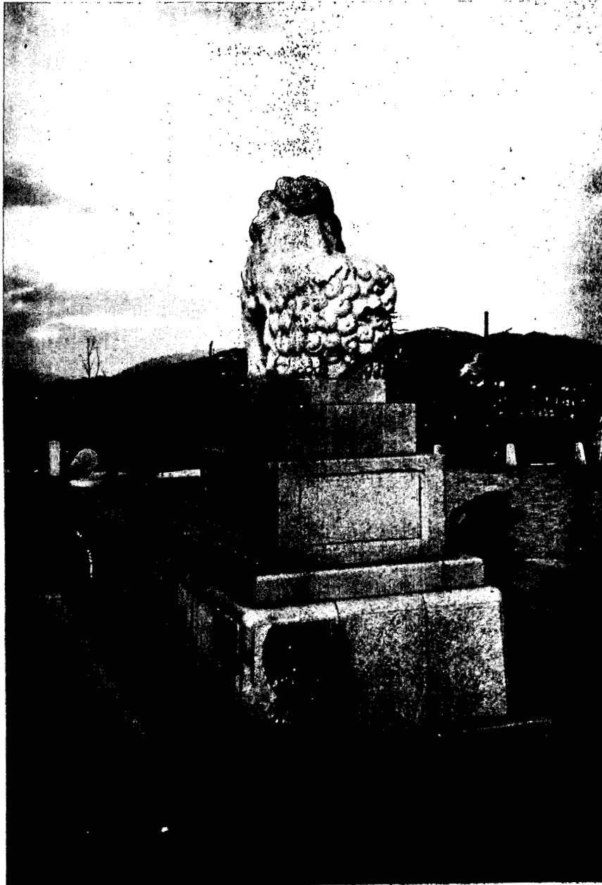
Fig. 14 (5H)--Gokoku Shrine (300 meters). General view of pedestal of a guardian dog at the shrine. The granite that was shaded retains its polish on the left side of the pedestal at the several levels; that which was exposed to the radiant heat is rough and light in color. This suggested to Japanese experts that at the surface of the granite, the temperature was as high as 2500°C. (Photo File #HE 108.)
