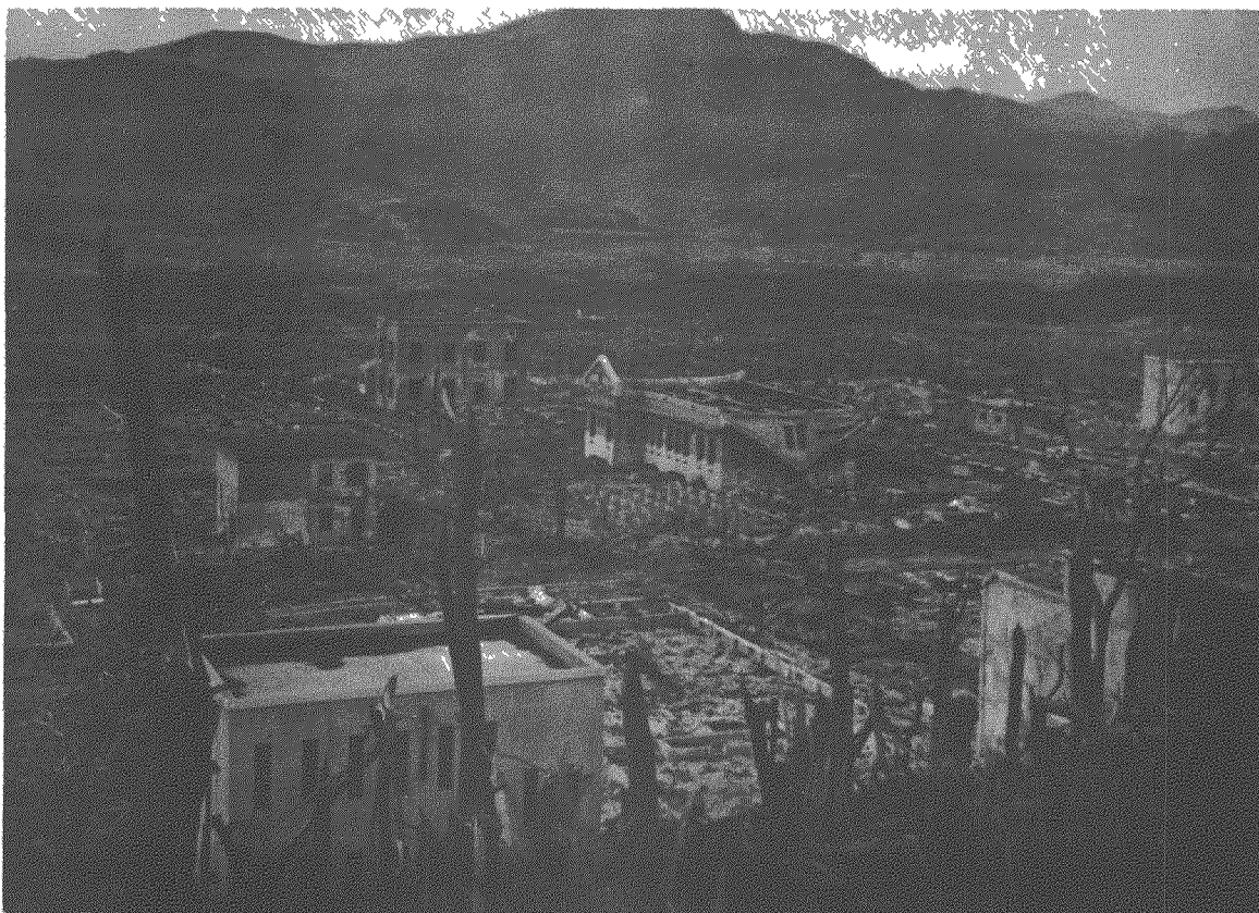
Fig. 20b--(3N). The buildings of the Nagasaki Medical College after the bombing. Only the reinforced concrete structures remain. (Photo File #NB 108c.)
