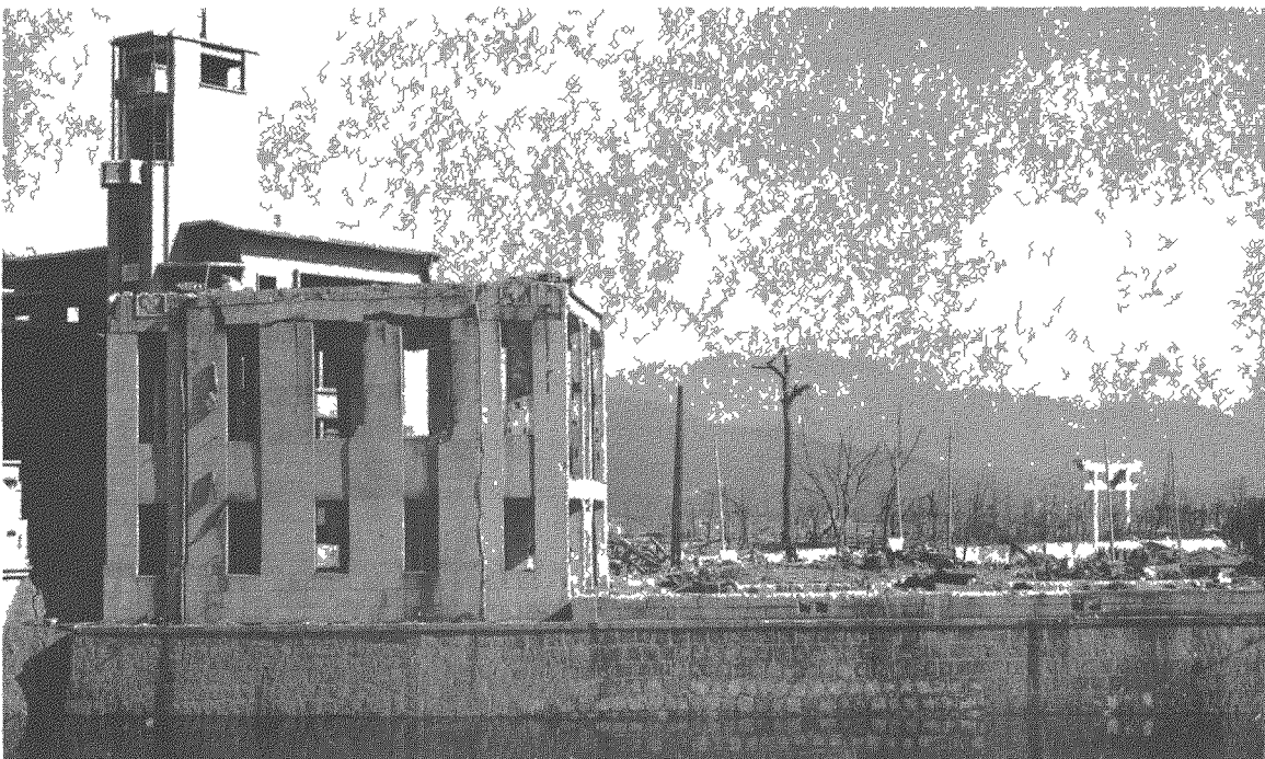
Fig. 14 a, b--(3H). Chamber of Commerce (300 meters) before and after the bombing. Complete destruction of the wooden building. Severe damage to the concrete structure. A new building ("Business-men's Club") has been constructed in the interval between the two photographs and looms at the rear. (Photo File # HB 115 a, b.)
