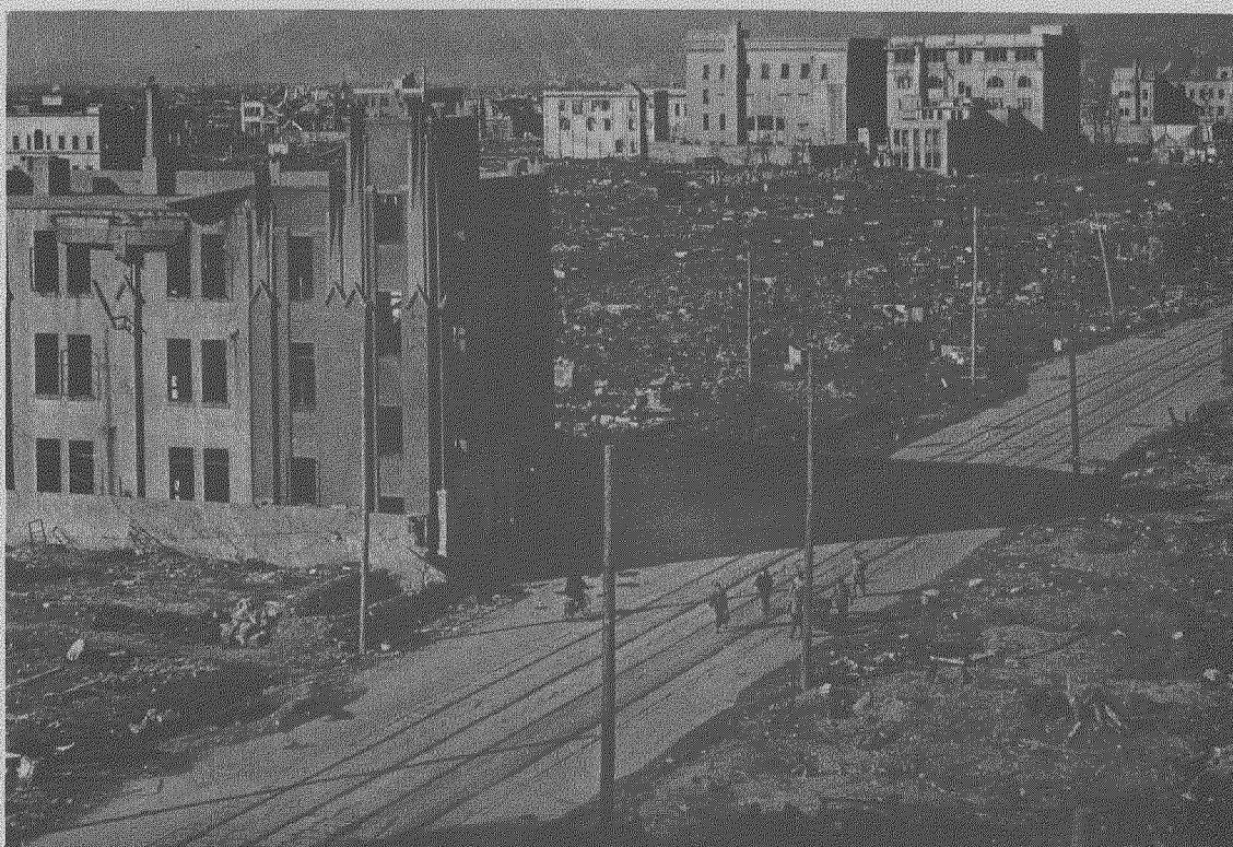
Fig. 9 a, b--(3H). Rear view of Geibi and Sumitomo Buildings before and after bombing. Taken from Fukuya Department Store (700 meters) looking toward center. Complete destruction of wooden buildings by blast and fire. Concrete structures stand. Note that parapet of the ecclesiastical structure in the foreground has fallen away from the center of the blast on the far side. The proximal parapet stands. This is probably the result of a blast reflection phenomenon. (See text.) (Photo File # HB 111a, b.)
