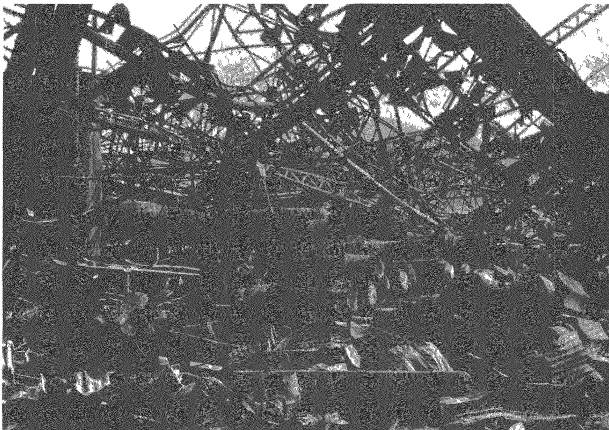
Fig. 12--(3N). Mitsubishi Steel and Arms Factory. Scene in one building where billets of steel for shells and guns were treated. This site is approximately 700 meters from the center. (Photo File #NB 437.)
