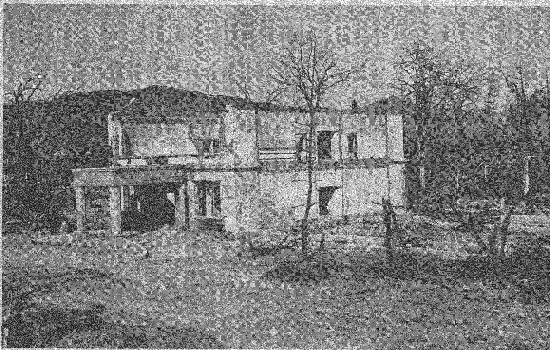
Fig. 16 a, b--(3H). Hqs. Chogoku Army (800 meters) before and after bombing. (A portico has been added since the first photograph). The wooden wings have collapsed and burned. The brick central section has partly collapsed. (Photo File # HB 113 a, b.)
