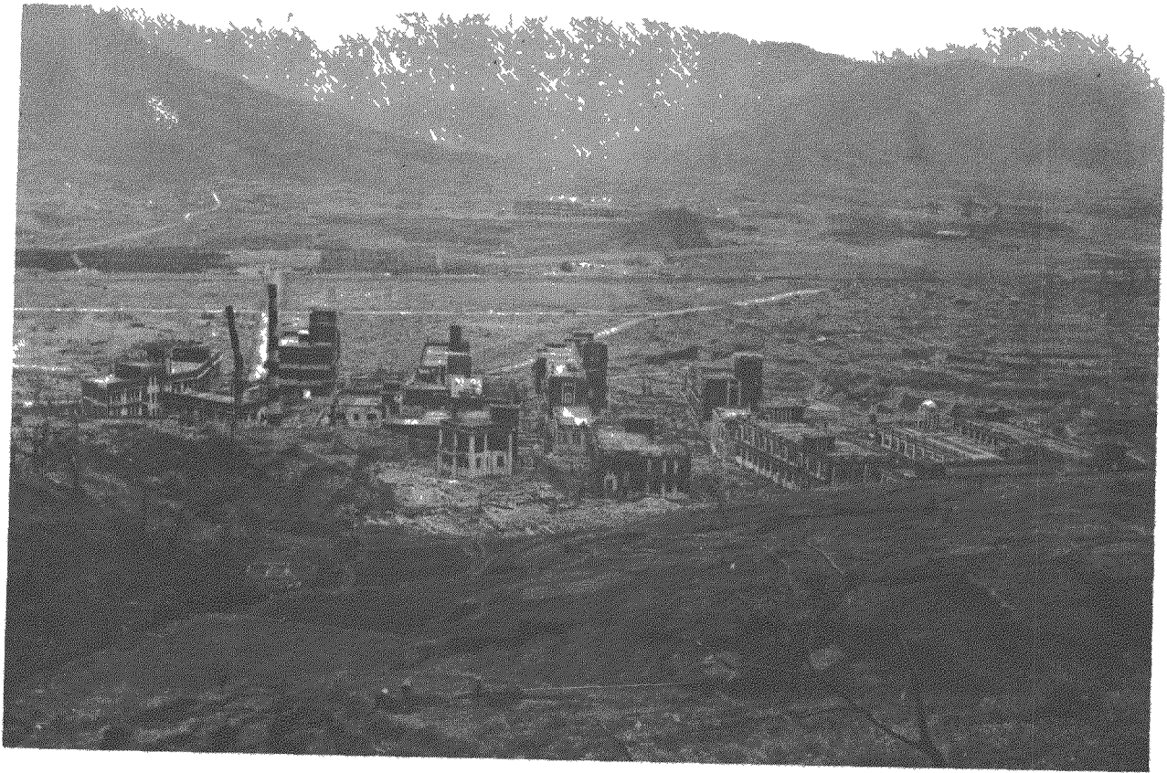
Fig. 18b--(3N). The Hospital of the Nagasaki Medical College after the bombing. Only the reinforced concrete buildings remain. (Photo File #NB 105b.)
