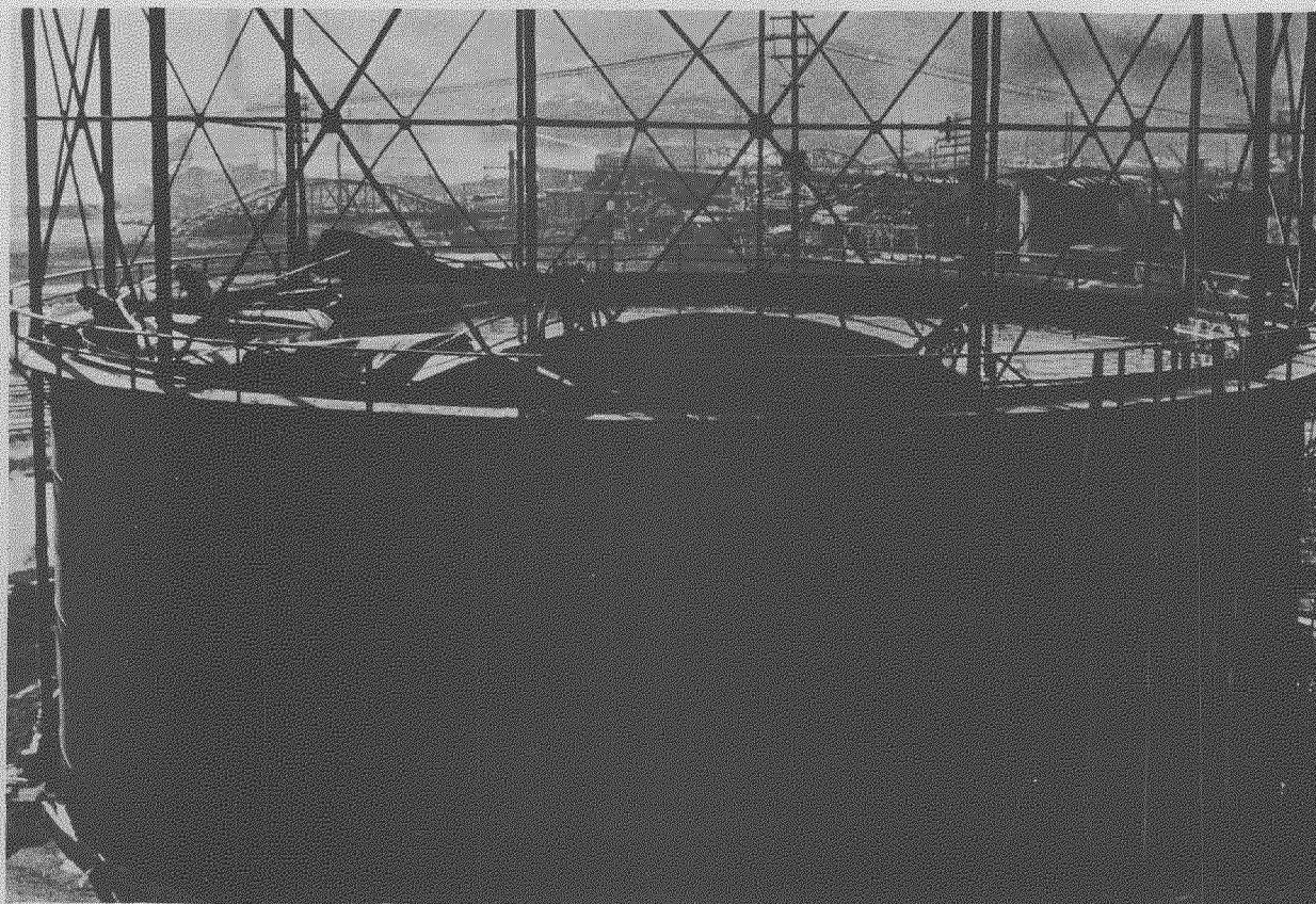
Fig. 14--(3N). One of two storage tanks of Urakami Gas Works, located 2,000 meters south of the center. The top is "dished" in by the blast but it is otherwise intact. (Photo File #NE 106.)
