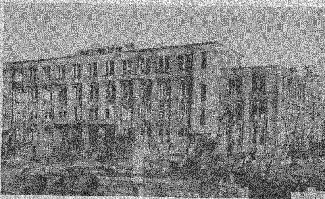
Fig. 13 a, b--(3H). Municipal Office (City Hall) (1100 meters) before and after the bombing. The "fire-proof" building has not suffered structural damage from blast, but suffered a disastrous fire. (Photo File # HB 102 a, b).
