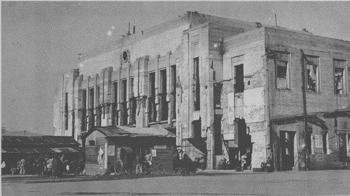
Fig. 12 a, b--(3H). Hiroshima Railroad Station (1800 meters) before and after bombing. Structure stands, but roof has collapsed (see figure 12 c). (Photo File # HB 105 a, b.)
