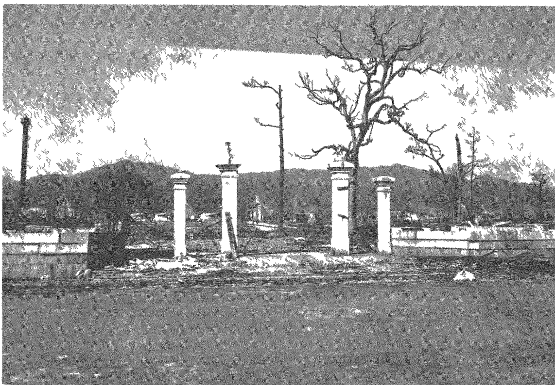
Fig. 17 a, b--(3H). Prefectural Office (900 meters) before and after bombing. The wooden structure has collapsed and burned. Note displacement of the heavy granite blocks of the wall. (Photo File # HB 112 a,b.)
