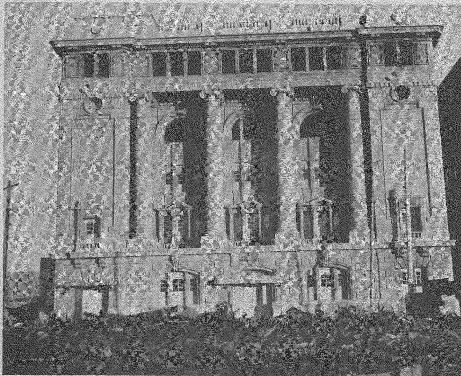
Fig. 11 a, b--(3H). Geibi Bank (250 meters) before and after bombing. This massive reinforced concrete structure withstood the blast but was swept by fire. (Photo File # HB 106 a, b.)
