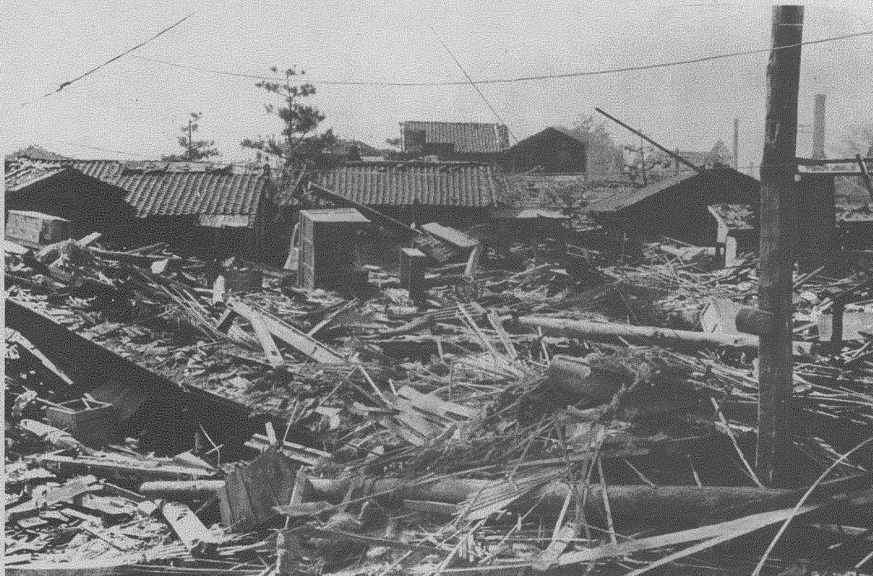
Fig. 20--(3H). Houses destroyed at Higashi-ura, Dunbara (2,000 meters). This area was partly protected from blast by Mount Hiji. The collapsed structures in the foreground represent the appearance of the city after the blast and before it was reached by the flames. The heavy tree beams were responsible for trapping many persons who were subsequently burned to death by the uncontrollable fires. (Photo File # HB 451.)
