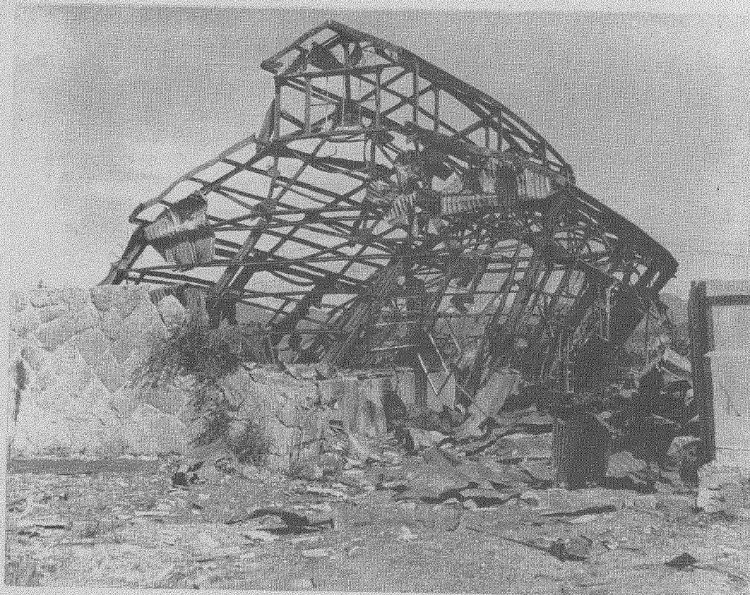
Fig. 19--(3H). "Mass distortion" of a steel-framed factory shed (600 meters). The entire building leans away from the center of the explosion. The metal sides have been crushed against the frame like paper blowing in the wind. (Photo File # HB 415.)
