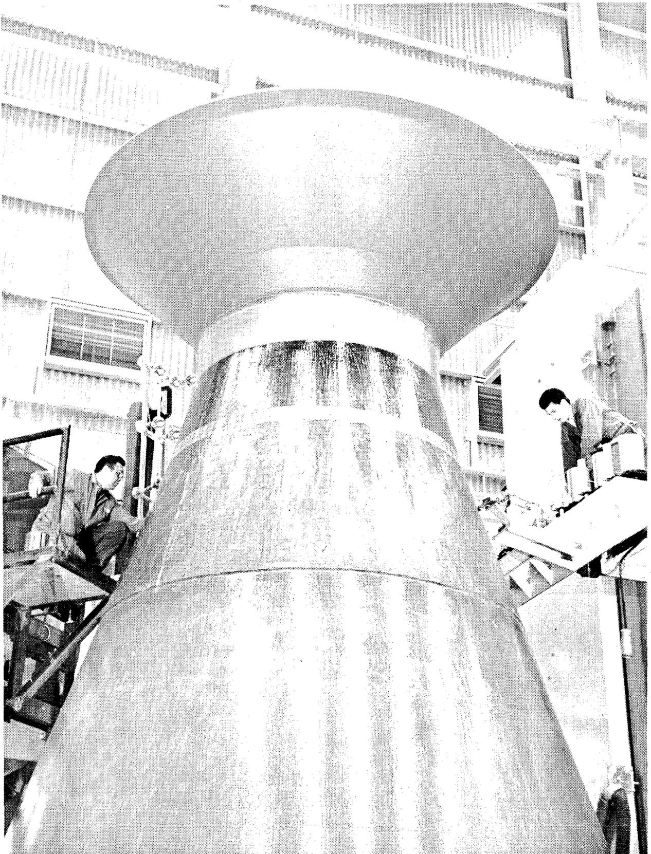
Figure 16 - Application of Tie Laminate
